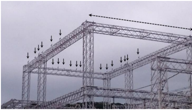
Figure 1. High Power Testing Laboratory of the Central Research Institute of the Electric Power Industry in Yokosuka, Kanagawa, Japan. Solid and dotted arrows represent grey herons landing on steel structures and the structure-attached LED light, respectively.
