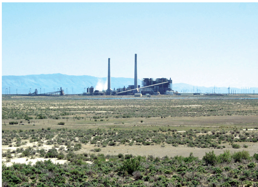
Figure 1. The Valmy coal-fired power plant in Humboldt County, Nevada.
