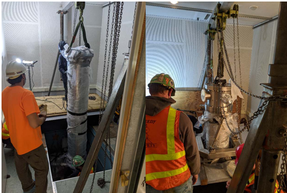
Figure 4.14: Images of the Sheedy workers during installation.
