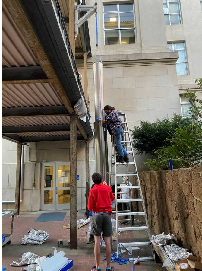
Figure 4.12: In case you ever doubted the strength of a single 1/4-20 bolt... The crane is attached to the I-beam with a single extreme strength 1/4-20 bolt from McMaster-Carr, though a thorlabs 1/4-20 bolt should have still had a large factor of safety.
