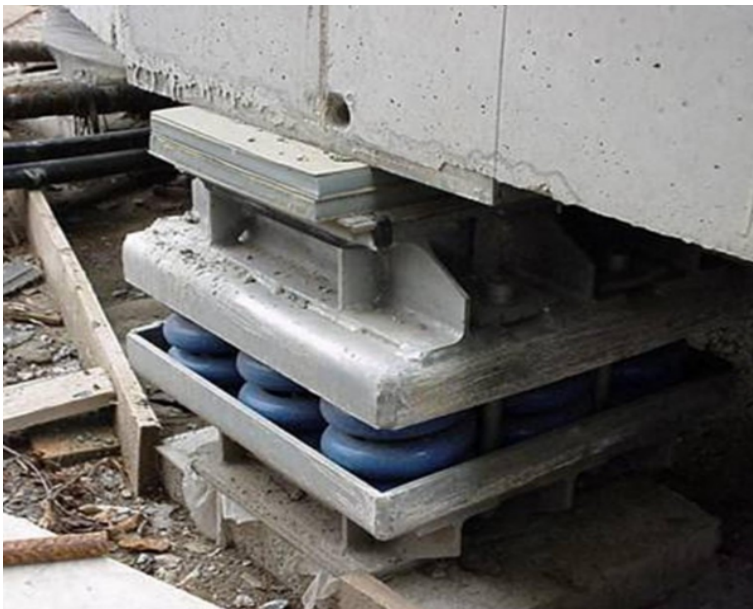
Figure 1.3: Steel spring bearings [18]
