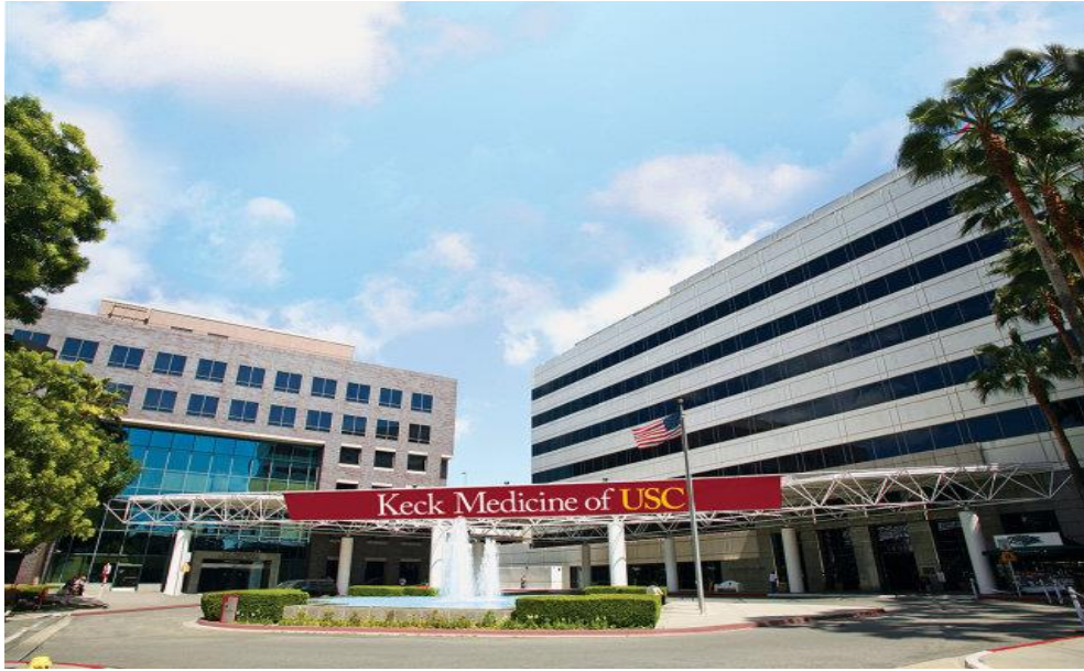
Figure 1.8: Keck Hospital of USC, Los Angeles, California, sits on 149 base isolators. Almost no damage was found on the main structure or the nonstructural components during the 1994 Northridge Earthquake [65].
