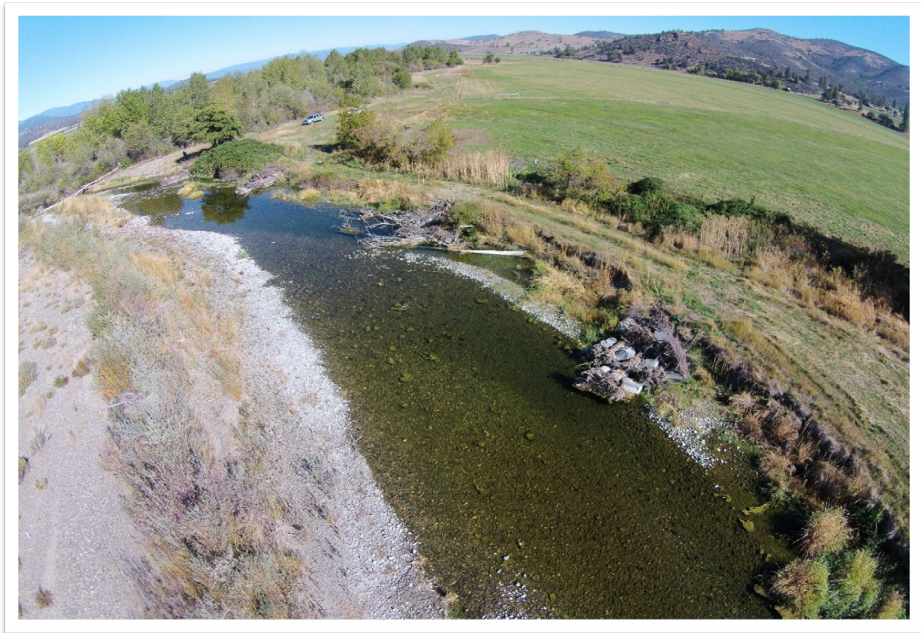
Figure 10. Large wood structures redirecting the flow from an eroding streambank. Photo credit: Joey Howard, Cascade Stream Solutions.
