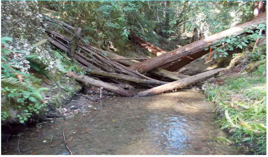
Figure 21. Logs pinned using threaded rebar. Photo credit: Chris Blencowe, Blencowe Watershed Management.
