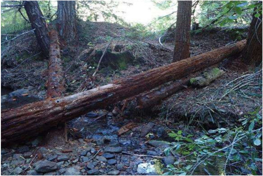
Figure 20. Logs wedged between trees and pinned at the apex for stability. Photo credit: Brett Leonard, California Conservation Corps.
