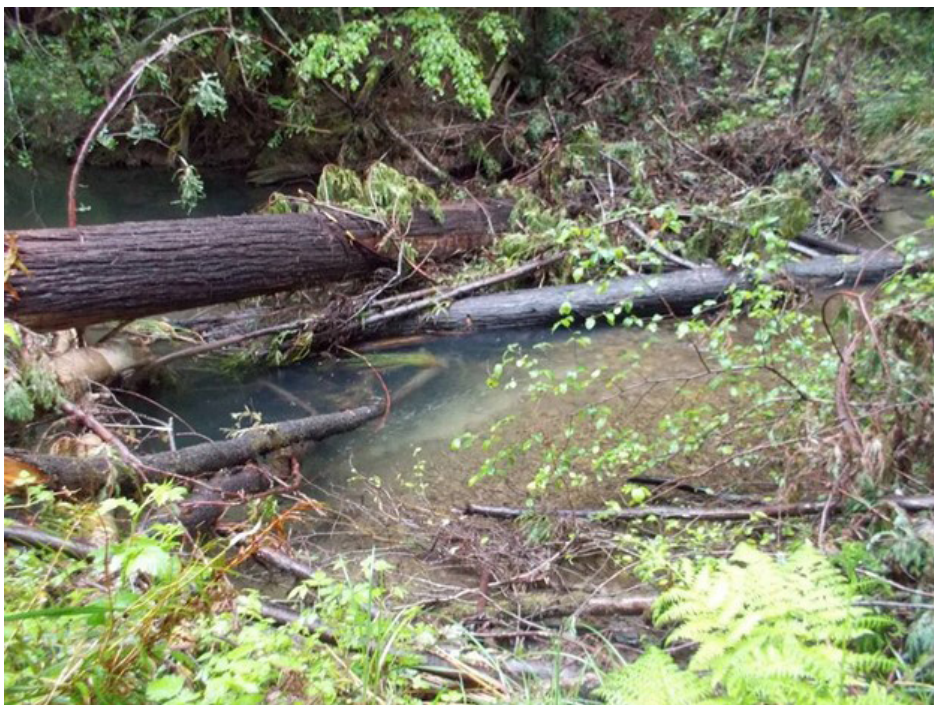
Figure 19. Felled key piece capturing woody debris with no added stability. Photo credit: Chris Blencowe, Blencowe Watershed Management.
