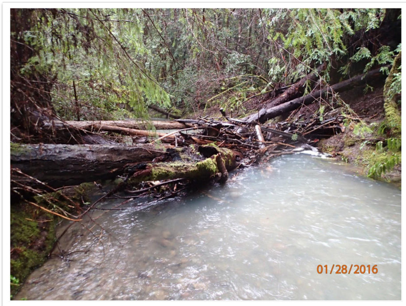
Figure 7. Additional woody debris collected by the structure shown in Figure 6 after the first winter in an active stream channel. Photo credit: Alan Ader, California Conservation Corps.
