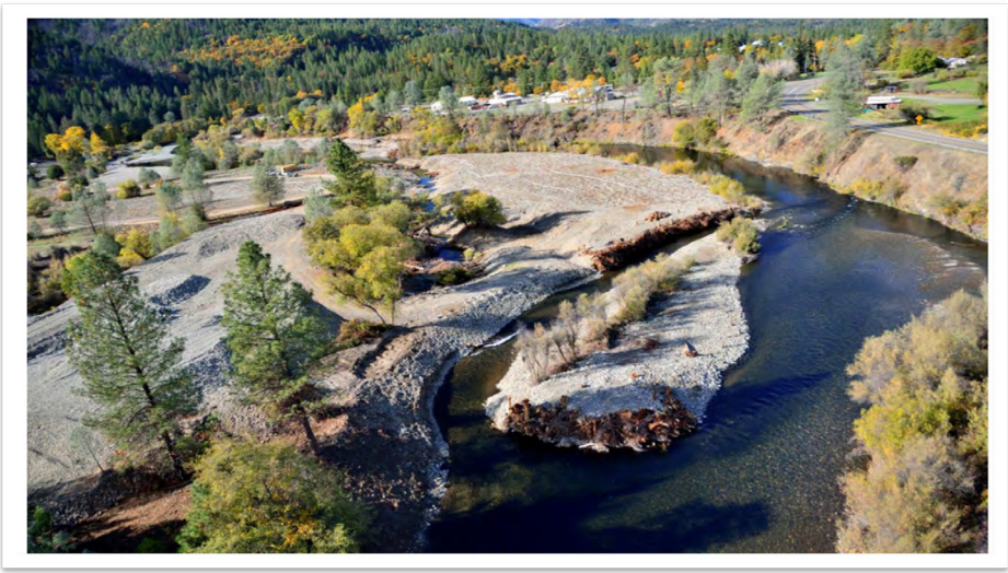
Figure 11. Apex bar jam redirecting flow into a side channel. Photo credit: David Bandrowski, Yurok Tribe.
