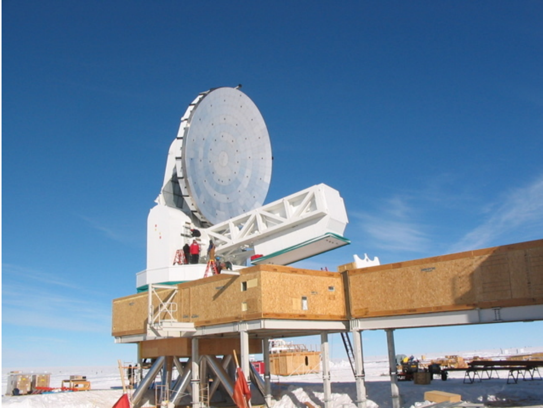
Figure 3.1. The South Pole Telescope during the last stages of construction, in the austral summer of 2006-2007. The large dish is the primary mirror, and the slightly elevated structure is the receiver cabin. During servicing and installation, the telescope is positioned so that the receiver cabin mates with the roof of the control room (right). The comoving ground shields were not yet installed when this picture was taken.
