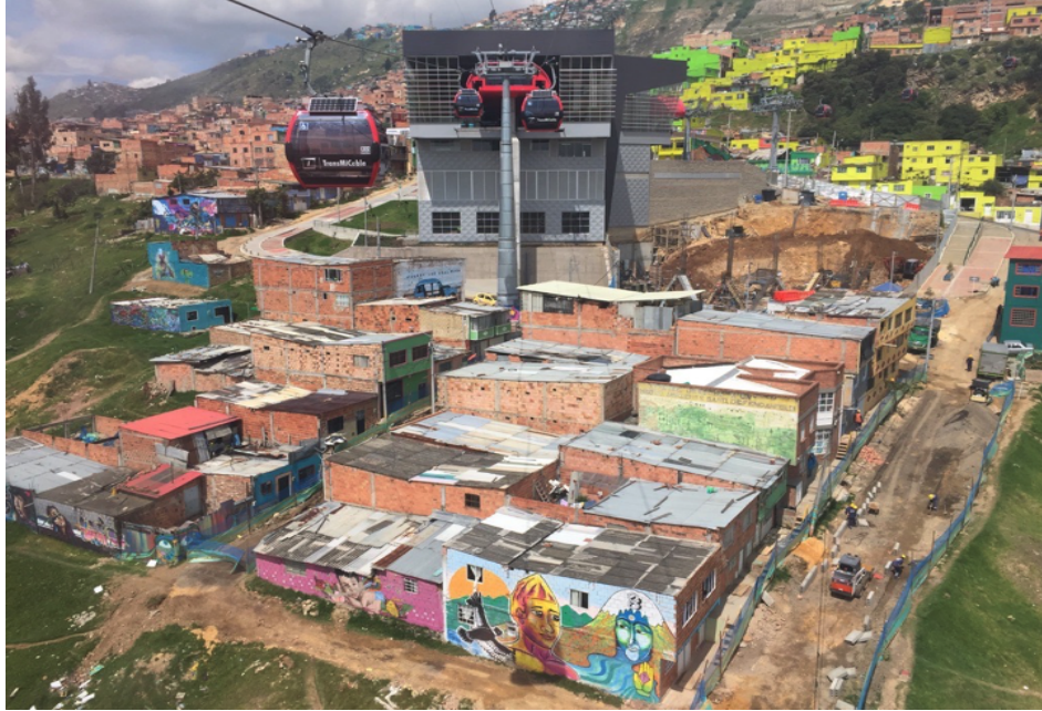
Figure 4-1 Arriving by TransMiCable to Manitas Station, in Ciudad Bolívar
