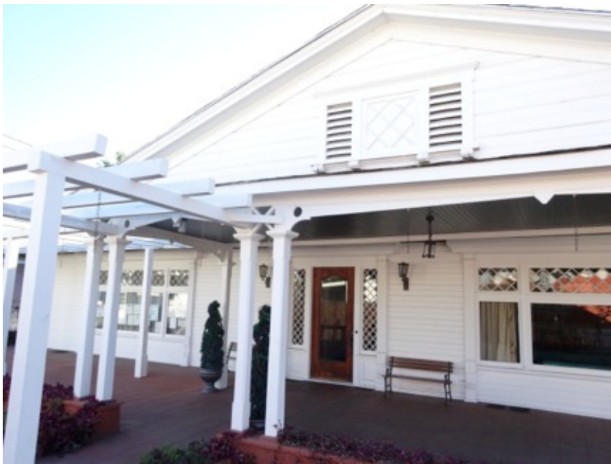
Figure 5. Front Entrance to Gage Mansion, Built Atop the Casa San Antonio, Bell Gardens, CA. Photo by Henry Grabar.
