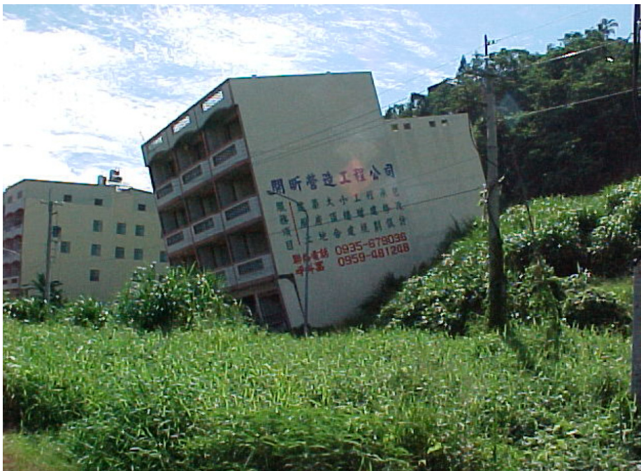
Figure 2-10. A building significantly rotated as a result of surface fault rupture during the 1999 Chi-Chi event (GEER 1999).
