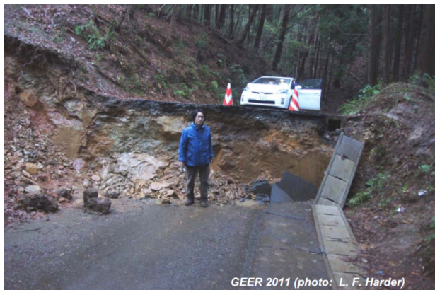
Figure 2-19. Free-field rupture from the 11 April 2011 Aftershock of the Great Tohoku Earthquake (GEER 2011).
