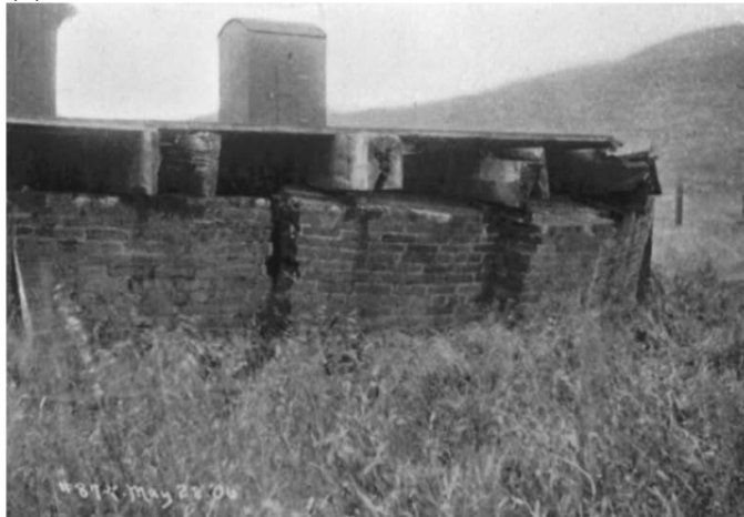
Figure 2-4. Fault rupture damages structures during the 1906 San Francisco Earthquake: (a) Plan view of the brick and concrete structures; and (b) the deformed brick forebay (Bray and Kelson 2006).
