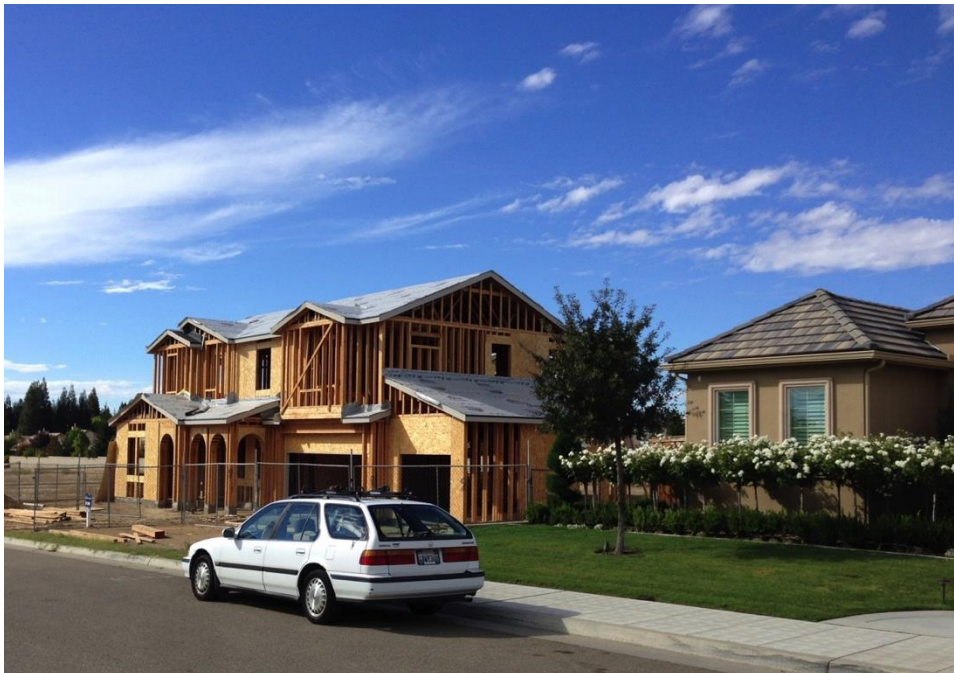
Figure 7 Fresno. Rough framing stage photo.
