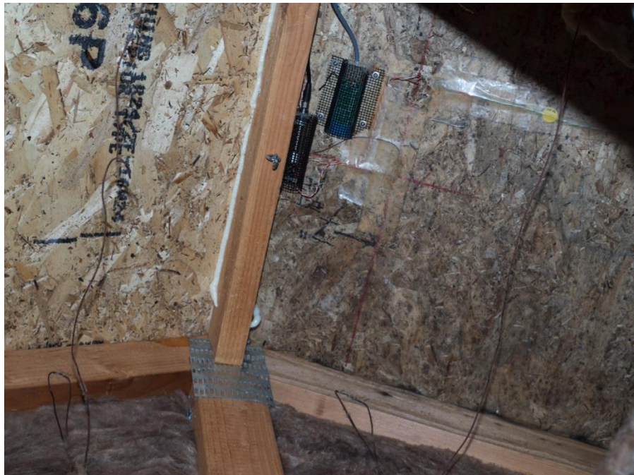
Figure 58 Clovis test home, photo of suspected mold growth on North-sloped OSB roof deck. Image shows location of monitoring equipment at the North slope ridge (right side), as well as the South sloped roof deck (left side) showing clean, unaffected OSB.
