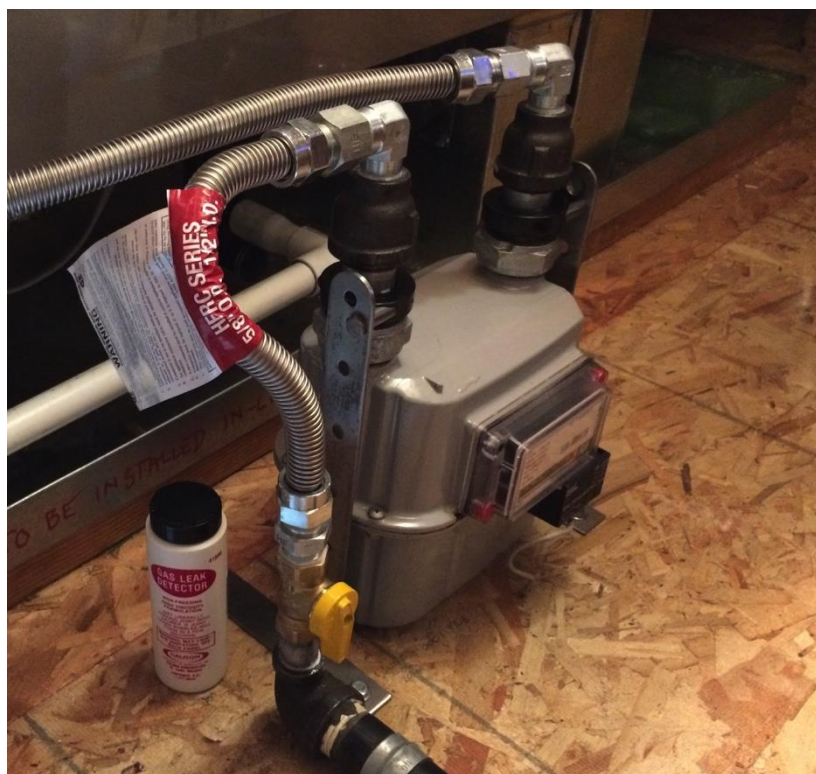
Figure 24 Gas sub meter with pulse output plumbed at natural gas furnace in Fresno attic.
