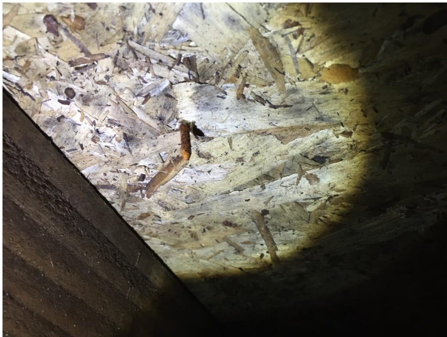
Figure 60 Clovis test home, photo of rusted roofing nail on North sloped roof deck.
