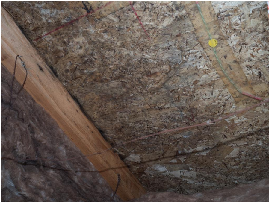
Figure 58 Clovis test home, photo of suspected mold growth on North-sloped OSB roof deck. Image shows location of monitoring equipment at the North slope ridge (right side), as well as the South sloped roof deck (left side) showing clean, unaffected OSB.
