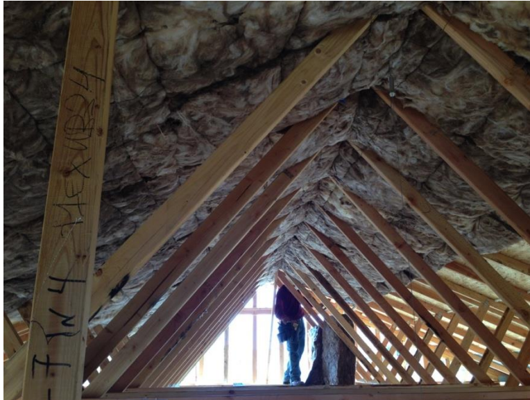
Figure 3 Image of R38 unfaced fiberglass batts installed with wire supports in the Fresno test home main attic.
