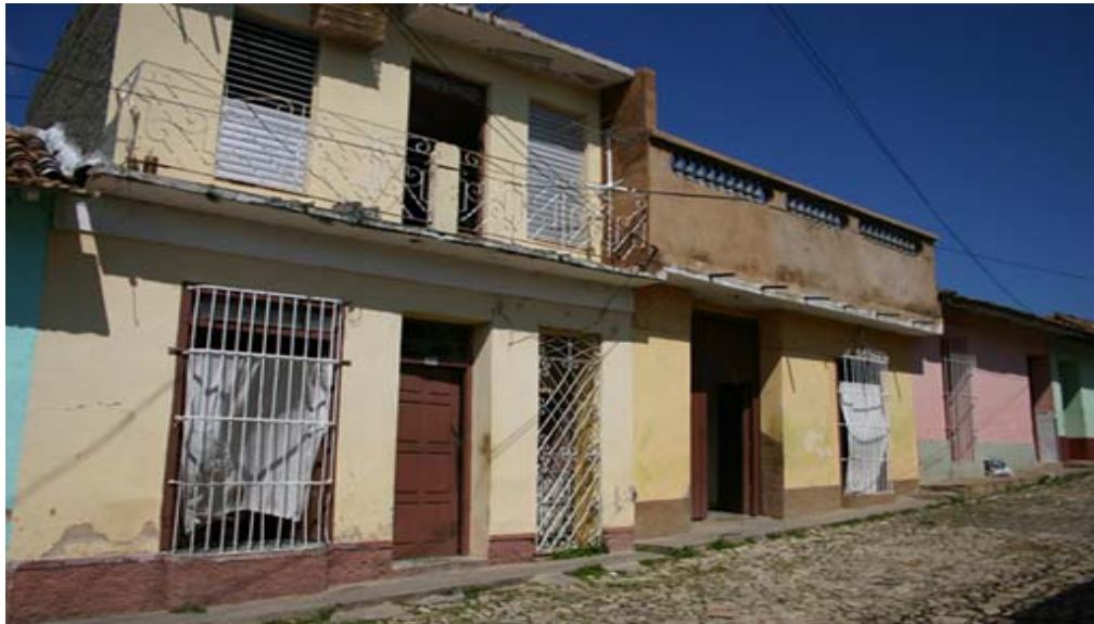
Figure 2.2 "Contamination": Restoration in violation of the building code. Photo by Maki Tanaka.
