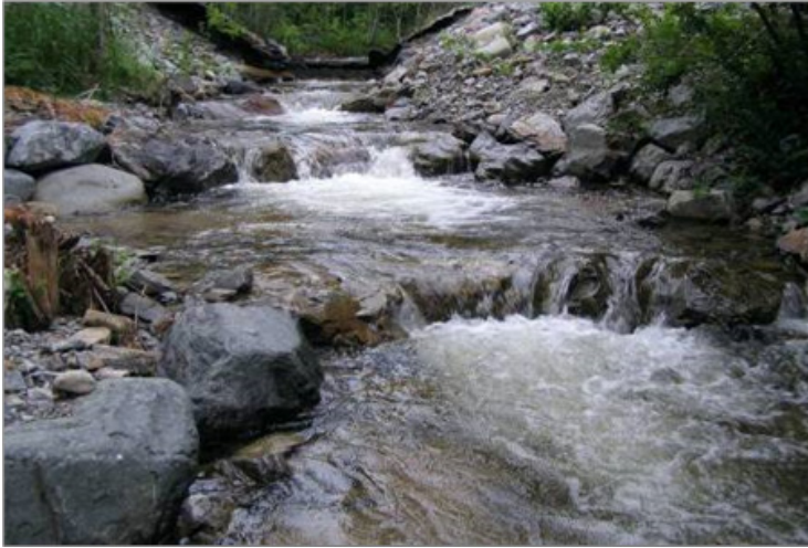
Figure 4. Arch-shaped boulder weirs produce diverse hydraulics across the crest while concentrating flow towards the channel center. Photo credit: Rob Sampson.
