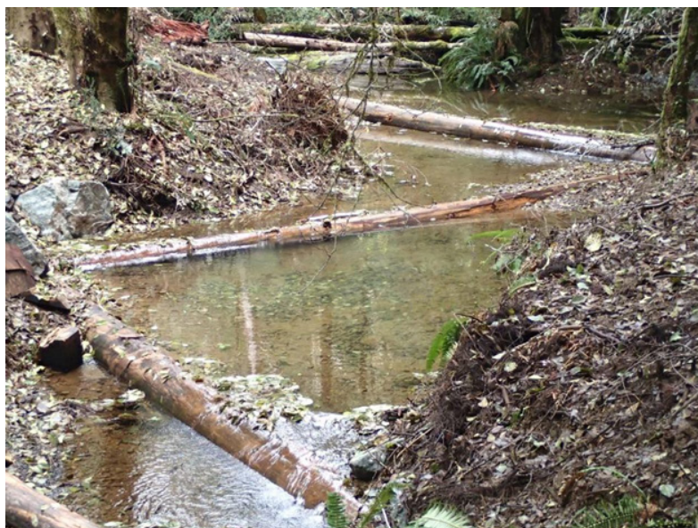
Figure 12. Diagonal log weirs in series. Photo credit: Sanctuary Forest.
