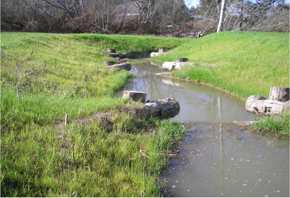
Figure 17. Series of log weirs with pilings as anchors. Photo credit: Mitch Farro.
