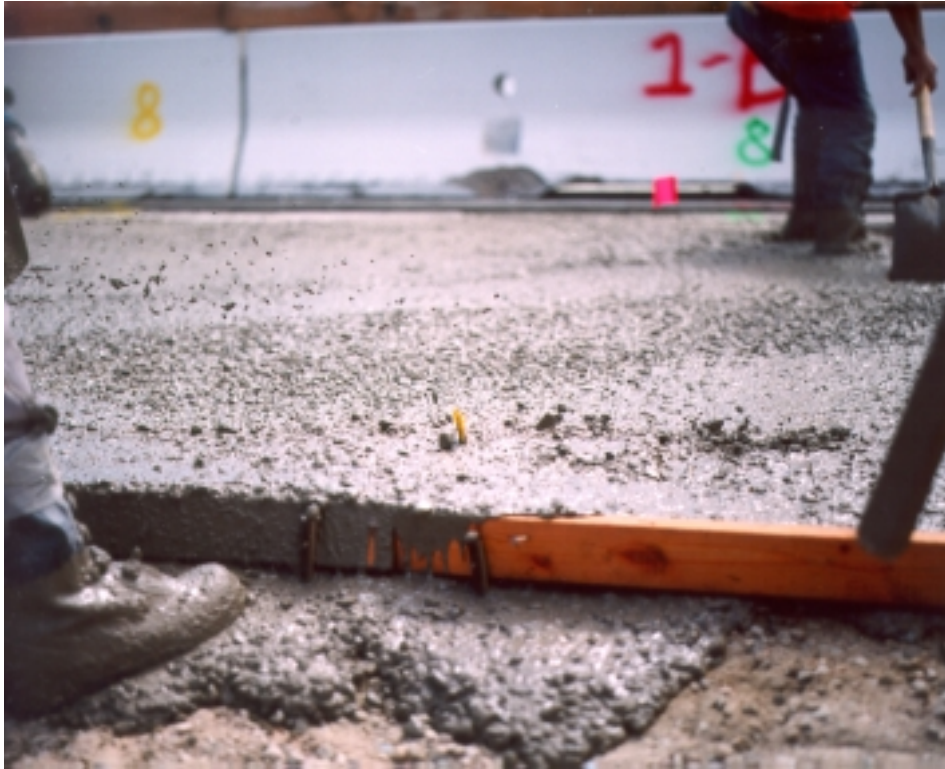
Figure 8.1. Wet Mix with Bleed Water on South Tangent.
