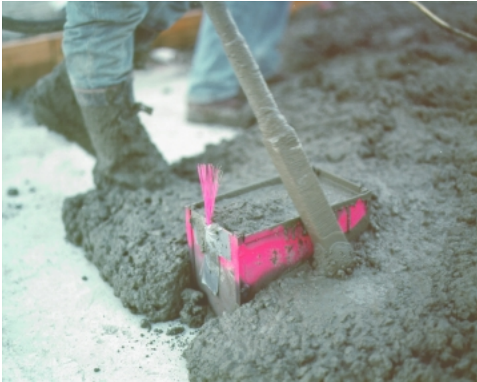
Figure 6.10. Vibrator Being Applied to Instrument Box to Consolidate Concrete.
