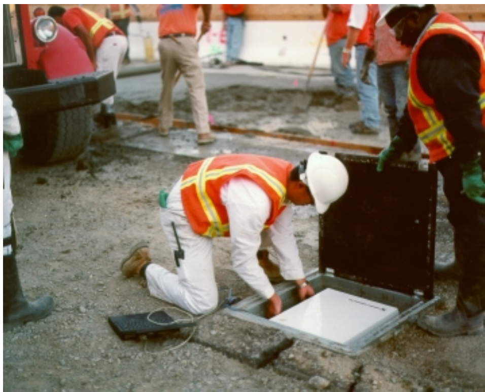
Figure 6.14. CR10X Acquisition System Being Placed on North Tangent.
