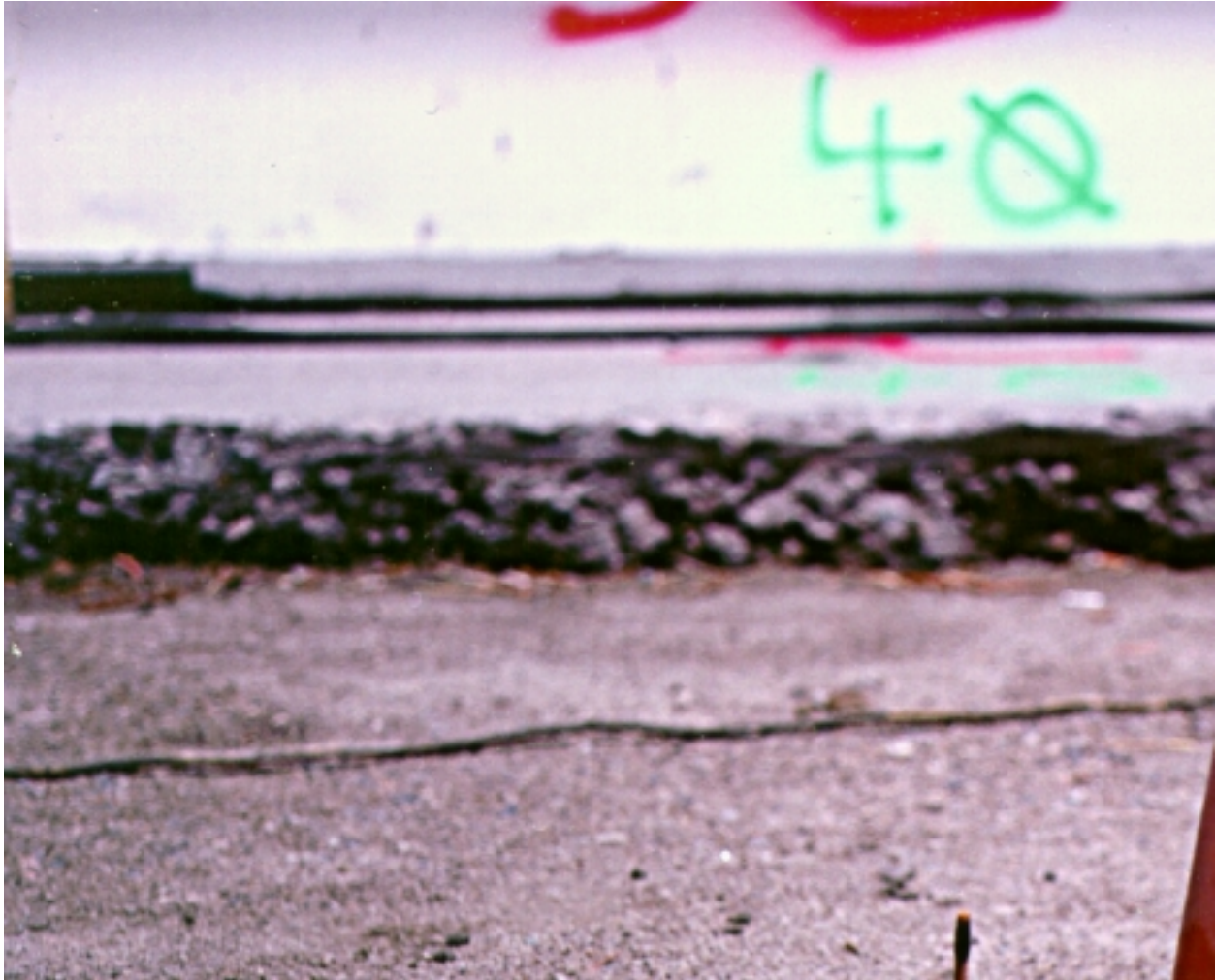
Figure 9.19. Detail photo of Rough Longitudinal Surface of Existing PCC Slabs, South Tangent.
