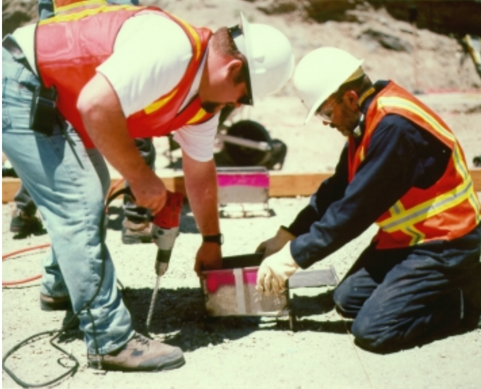
Figure 6.6. Steel Instrument Box Being Installed on South Tangent.
