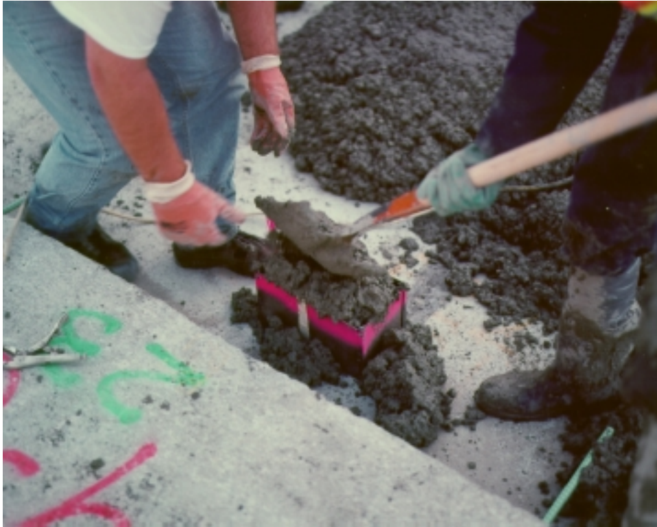
Figure 6.9. Instrument Box Being Filled by Shovel, North Tangent.
