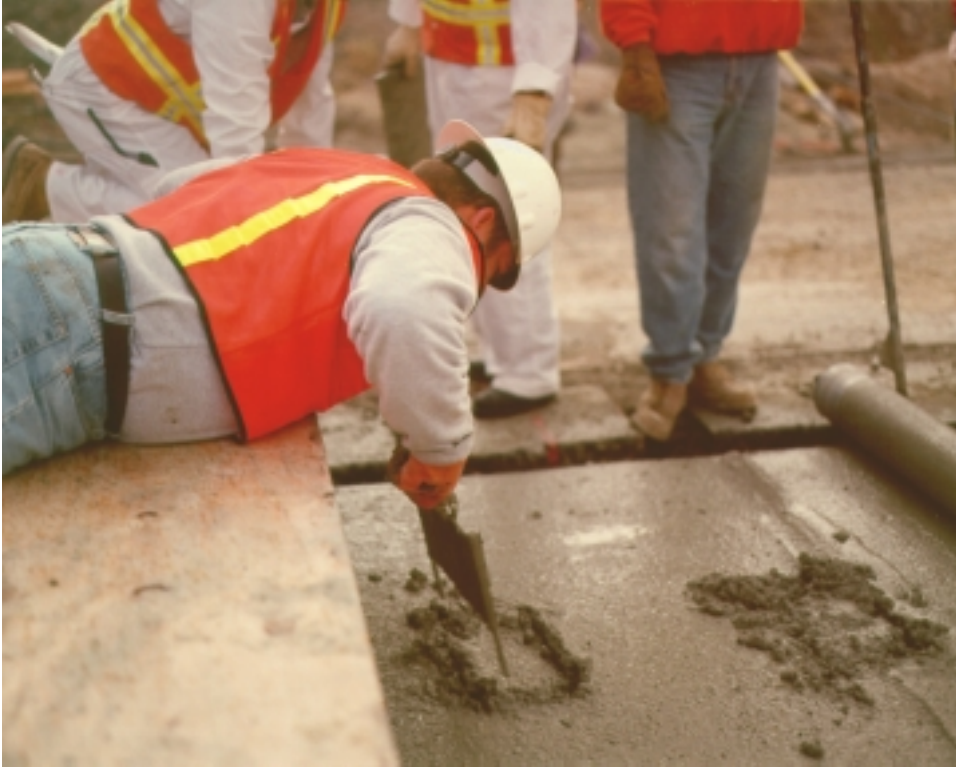
Figure 6.11. Technician Lying on Bridge over Test Section Removing Instrument Box.
