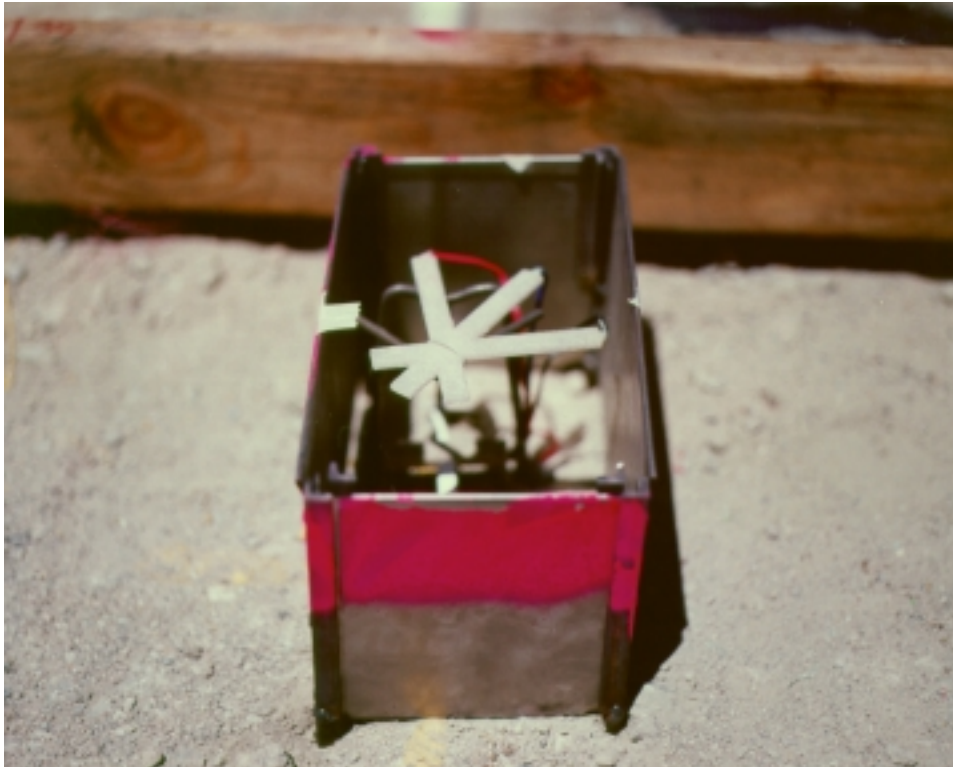
Figure 6.7. Steel Instrument Box Protecting Strain Gages on South Tangent.
