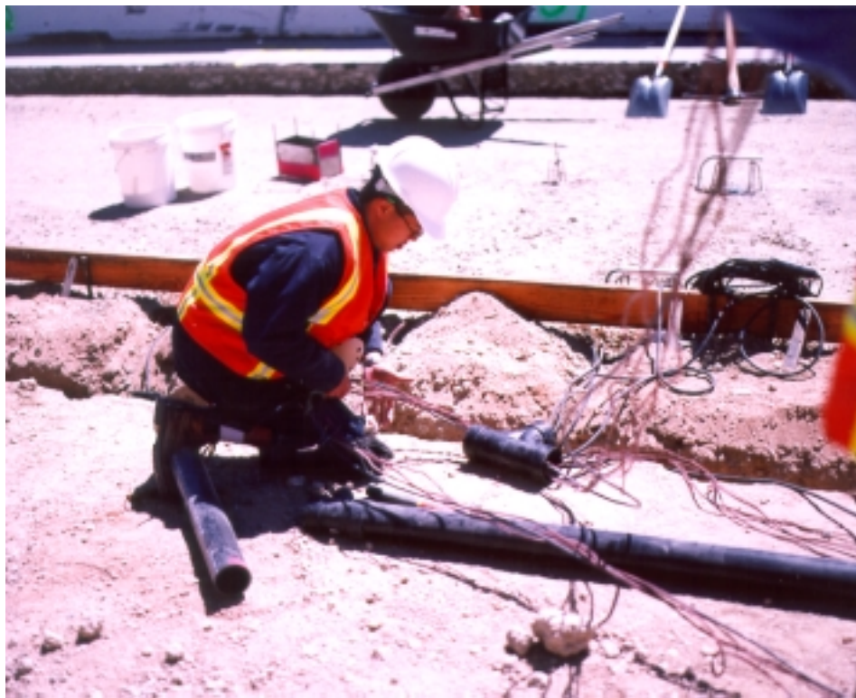
Figure 6.1. South Tangent Instrument Wiring and Piping Laid in Aggregate Base.
