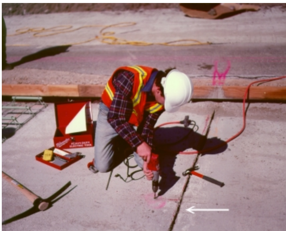
Figure 6.2. Grooves cut in North Tangent CTB for Instrument Leads.
