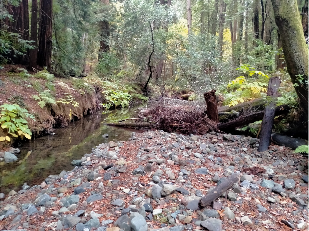
Figure 10. Downstream view of the river approximately at station 5650 ft with LWD4 on the right and undercut bank on the left in the place where riprap L10 was removed.
