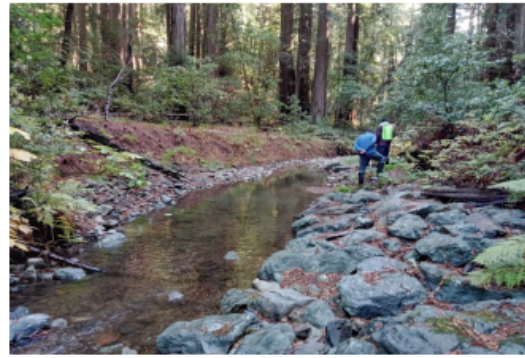
Fig. A5.4: View upstream, post-project
