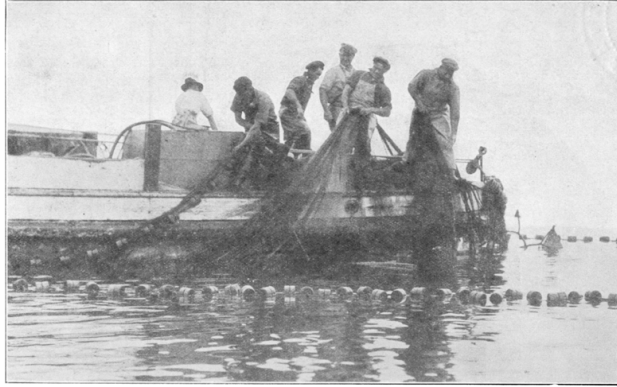
FIG. 1. Hauling a mackerel ring net. The purse rings can be seen bunched at the stern of the boat. July, 1929.
