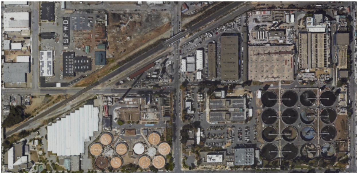
Figure 13: Southeast Pollution Control Plant in San Francisco (Source: Google Earth).
