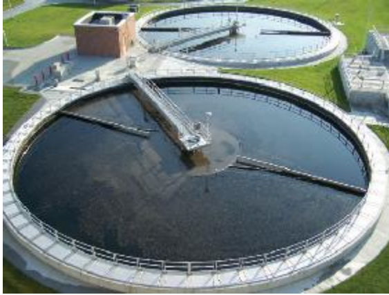
Figure 7: Example primary clarifiers.
