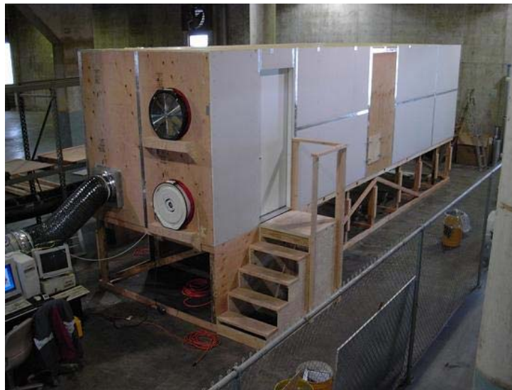
Figure 1. Completed test chamber inside warehouse showing the return duct connection and blower door fans, but before supply duct installation.
