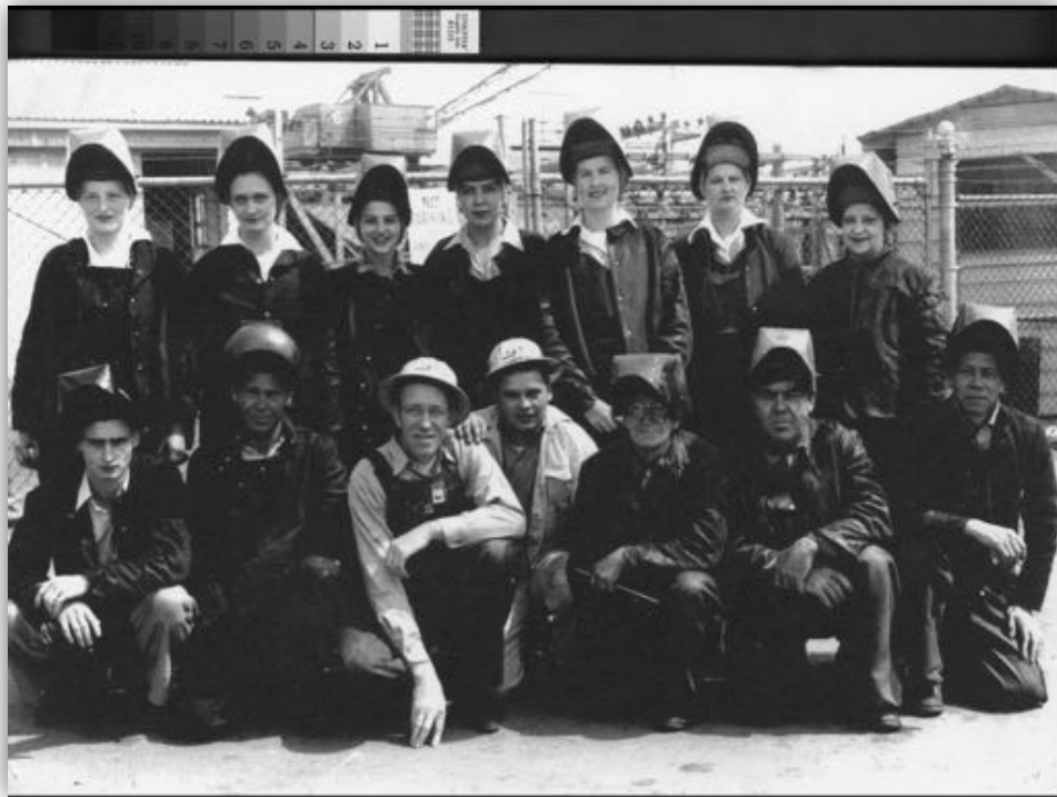
Figure 26. Welder Crew at the Kaiser Richmond Shipyards. Image courtesy of Richmond Museum of History.
