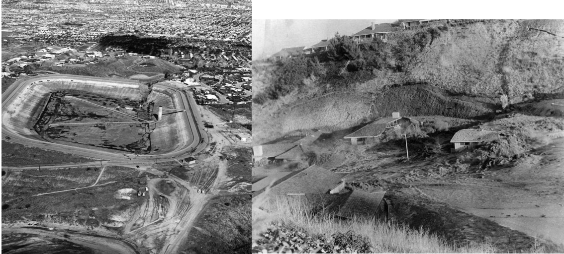
Figures 42-43: The Baldwin Hills Reservoir and floodwaters after the dam collapse in 1963
