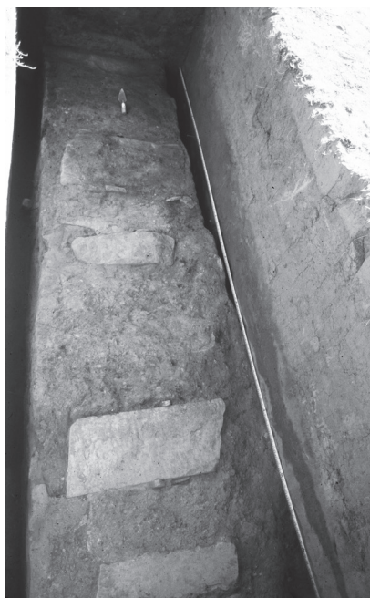
Figure 6.6 View of the top of the canal in Unit 6.23, stones and dark clay sealant intact.
