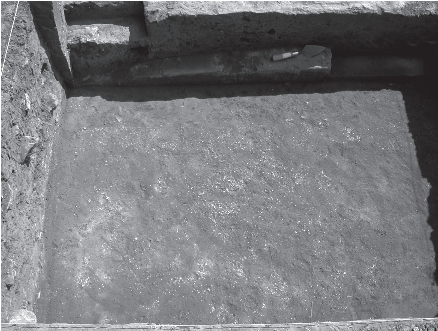
Figure 7.10 View of the floor near the west wall showing plaster flakes.
