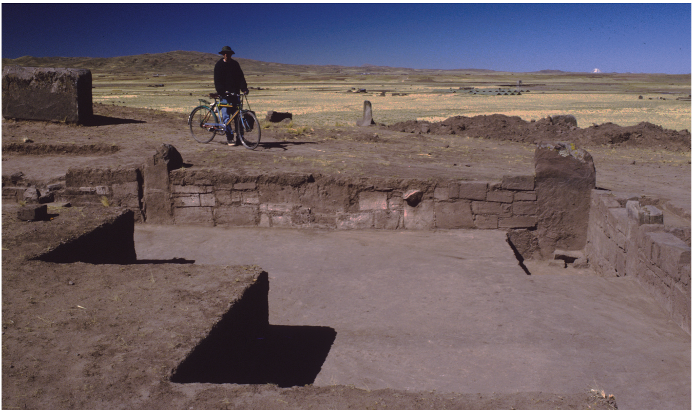
Figure 7.5 (below) View of the excavated southwest corner of the Sunken Temple, facing south.
