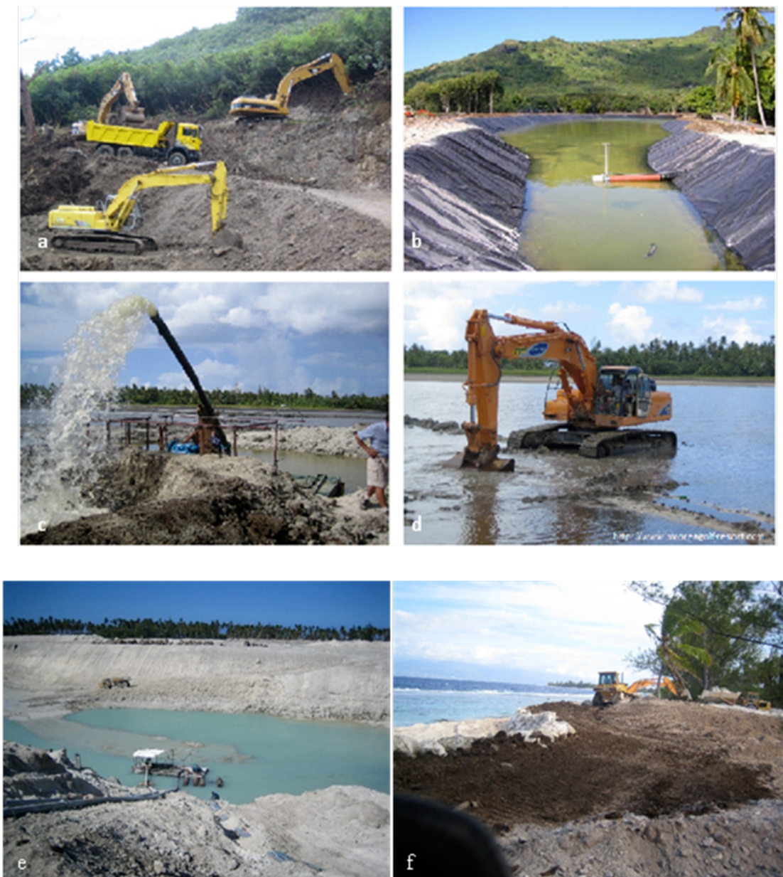
Fig. 7. Beginning stages of golf course development. Terracing (a), future golf ponds (b), draining, filling, and reshaping of Lake Temae and wetland(c) and (d), filling of “new” lake (e), and coastal development (f). 2005-2006 Source: Moorea Golf Resort website ( http://www.moorea-resort.com )
