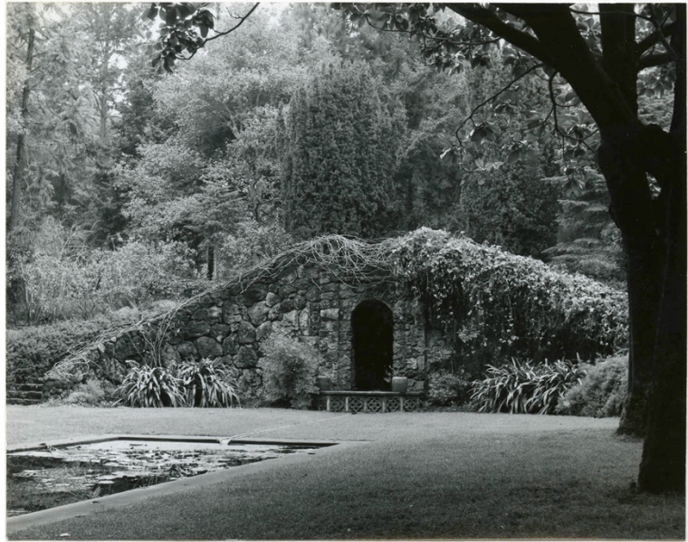
Figure 2: At the Anson and Anita Blake garden Symmes employed a classical approach opposite the front of the house, capturing a small creek to create a grotto within a retaining wall. Twin stairs behind the wall provide access to the hill. A rectangular reflecting pool completes the scene. Undated photo. Anson and Anita Blake garden, Blake Estate Collection, Environmental Design Archives, UC Berkeley.
