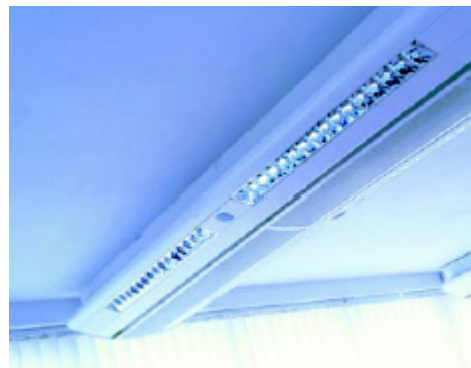
Figure 8. Chilled beams have been installed in laboratories in Europe and are beginning to be applied in the U.S. as well. Source: TroxUSA
