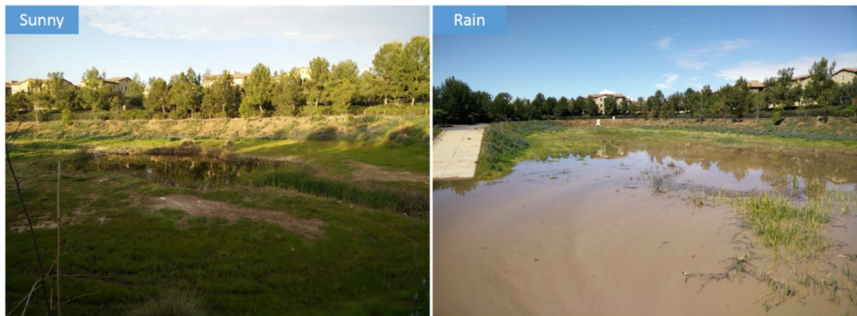
Figure 3-6 Constructed stormwater wetland (Forge) during sunny and rainy days. The wetland was inundated after a moderate rain (1.47 cm).
