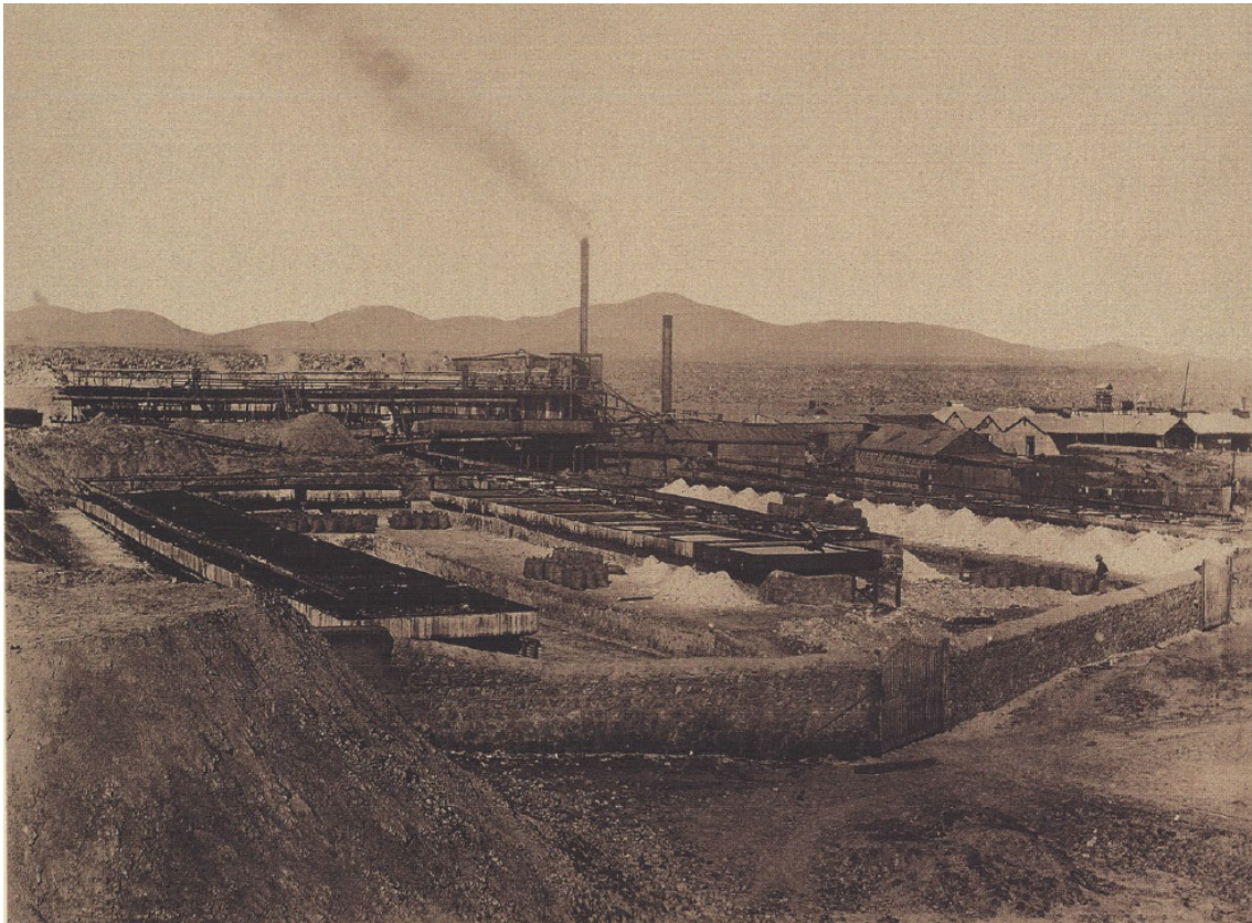
Figure 2.2.1: Nitrate Plant Example: Bearnes Plant
