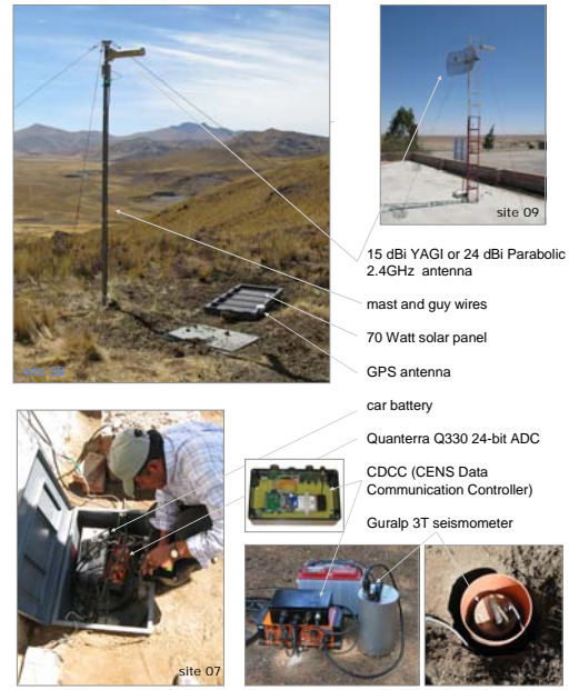
A typical site installation.
