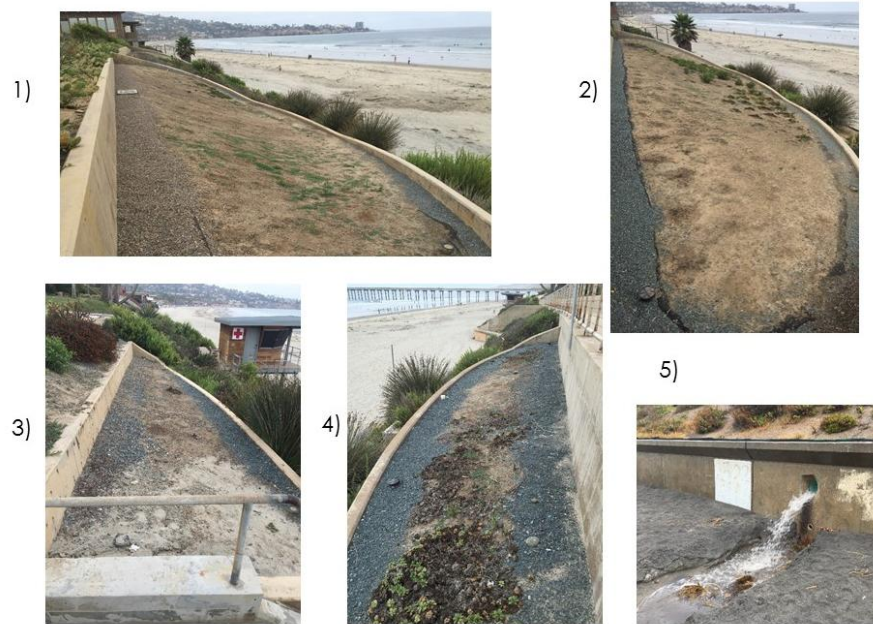
Figure 3- Pictures of the SIO biofilters. From top left: 1) TC-02, 2) TC-02, 3) TC-03, 4) TC-04 and 5) outfall onto the beach.
