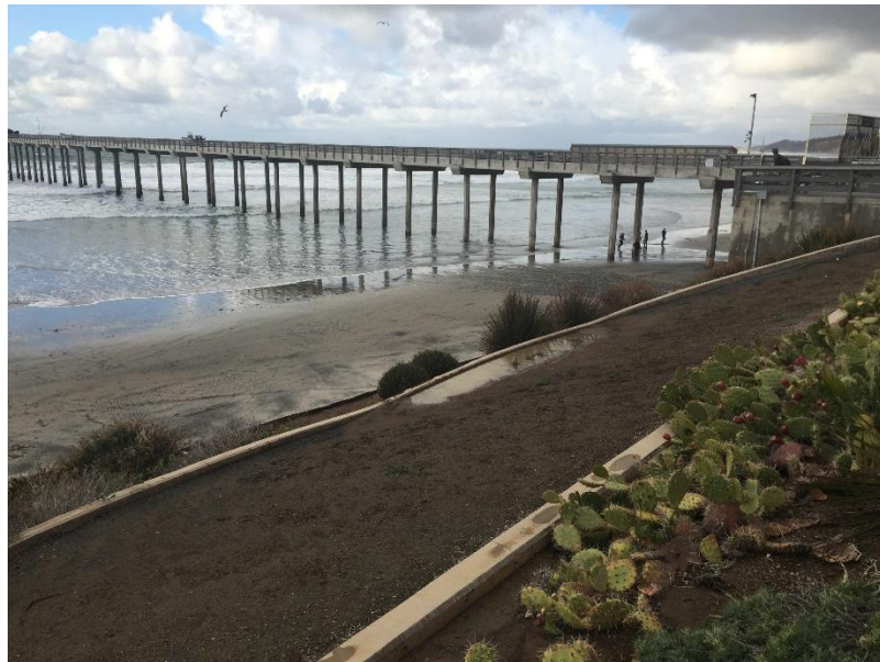
Figure 12 - TC-01 Flooded on January 7, 2016
