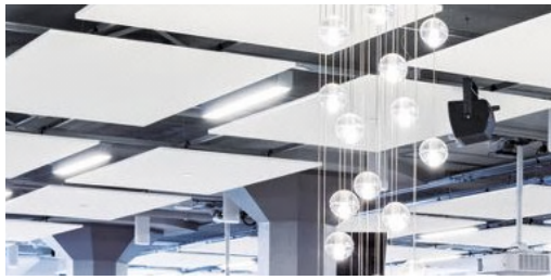
Figure 15: (Left) Example of free-hanging acoustic clouds (image: Armstrong World Industries); (Right) Section schematic of a ceiling with acoustic clouds and ceiling fan in upward and downward blowing directions
