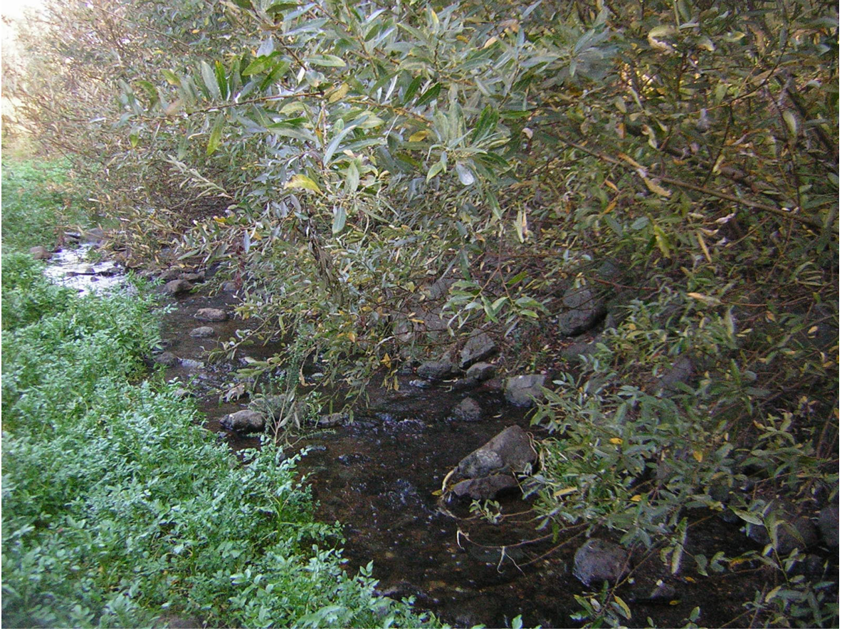
Photo 20: The last 100 feet of the site contains a long, continuous riffle. The vortex weir that was installed near this location here may be buried, or it may have broken up. We observed a number of appropriately sized rocks, but not in a vortex weir shape.
