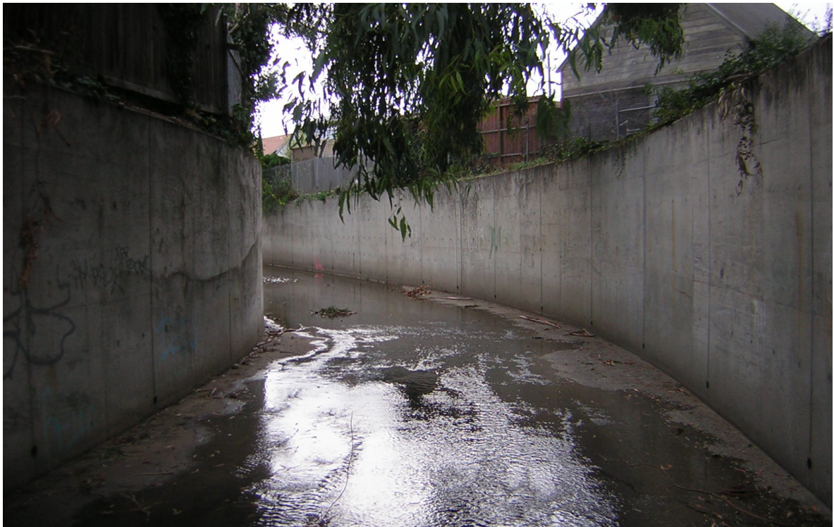
Photo 21: Downstream of the project reach, Arroyo Viejo creek is channelized and devoid of vegetation.
