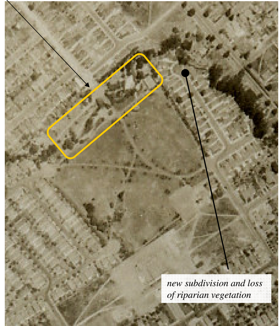
Figure 3b: Aerial Photo, 1946
