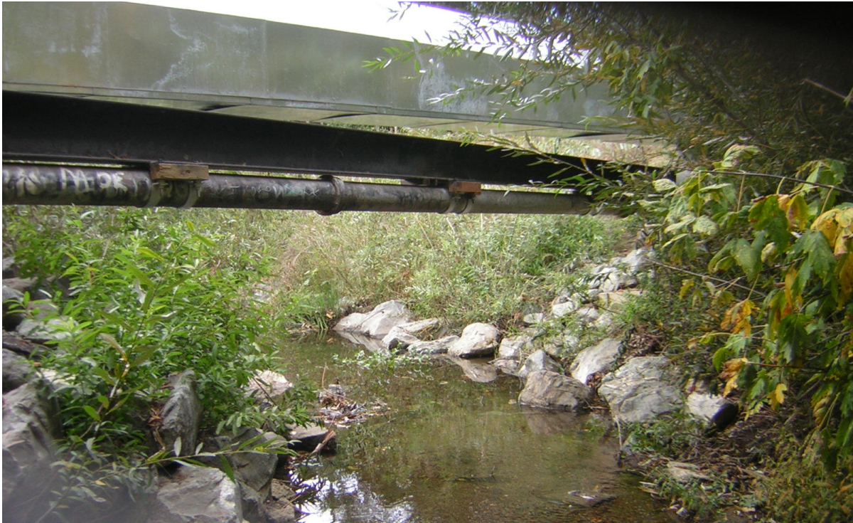
Photo 3. Looking west from the eastern end of the Project site, near the location of cross section A-A'. Utilities (not identified on the design documents) were protected and concrete rip rap was added to minimize scour-induced erosion of the stream bank. Vegetation growth can be seen through the placed rip rap boulders.
