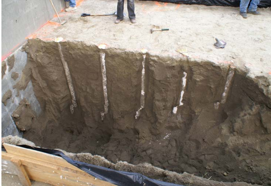
Figure 6.5. Exposed gypsum columns
