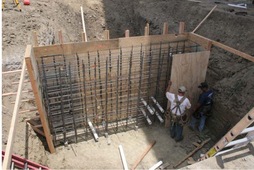
Figure 4.2. Reinforcement configuration in test specimen
