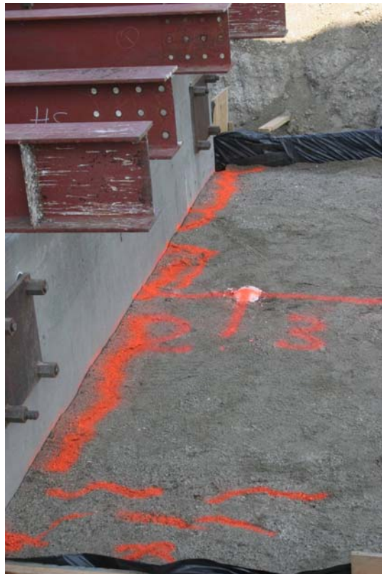
Figure 6.3. Photograph of crack patterns along the wall
