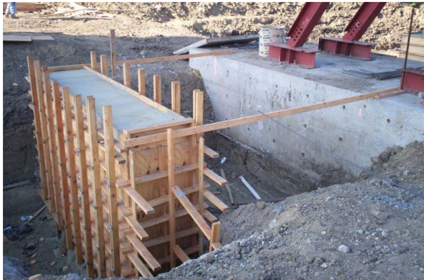
Figure 4.3. Photograph of wall after concrete pour
