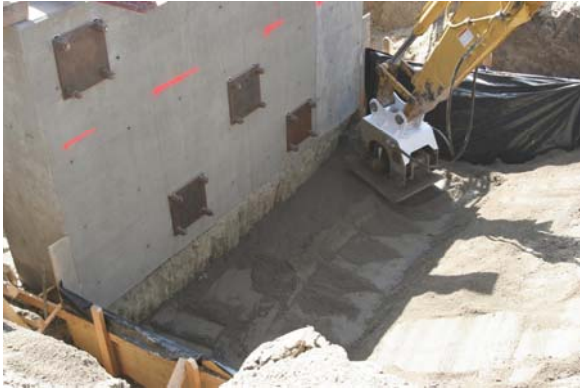
Figure 4.7. Vibratory compaction of backfill soils
