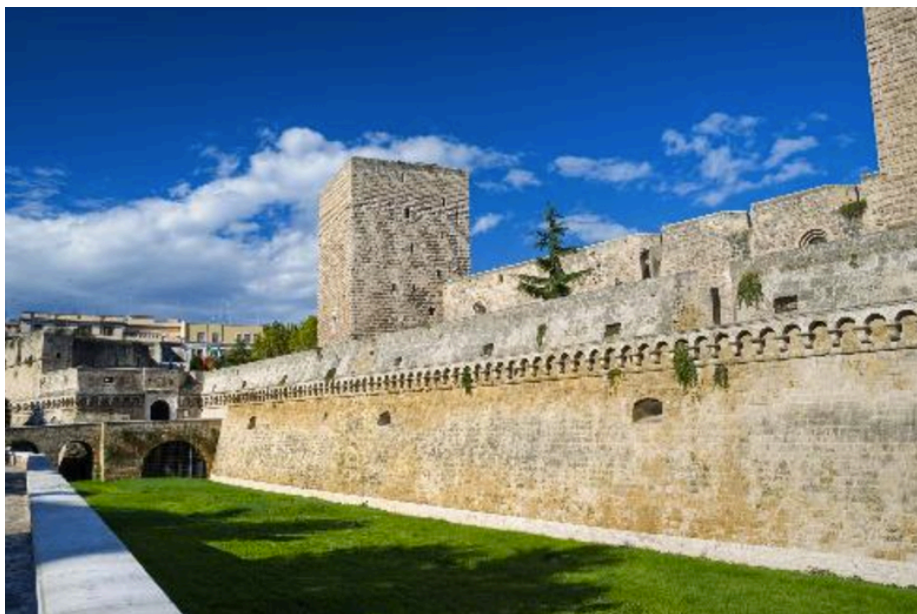
Fig. 3-14: The Swabian Castle (Castello Svevo) in Bari, built in 1131 by King Roger II of the Norman kingdom of Sicily and rebuilt by Frederick II, king of Sicily and Holy Roman Emperor, in the 1230s. 573
