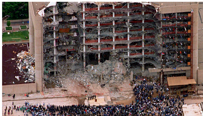
Figure 1.1: The Alfred P. Murrah Federal Building after bombing
