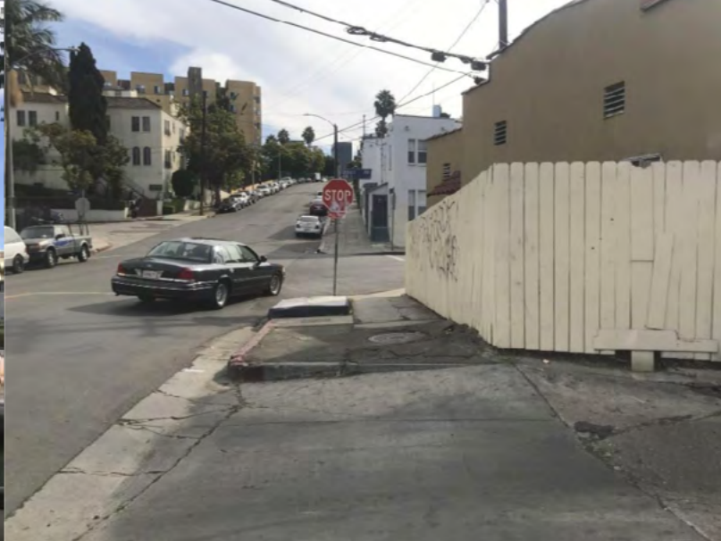
Figure 28: Cracks and uneven pavement
