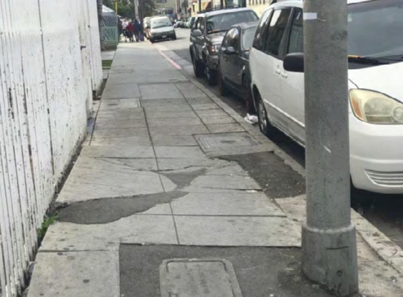
Figure 29: Cracks and uneven pavement on walking route
