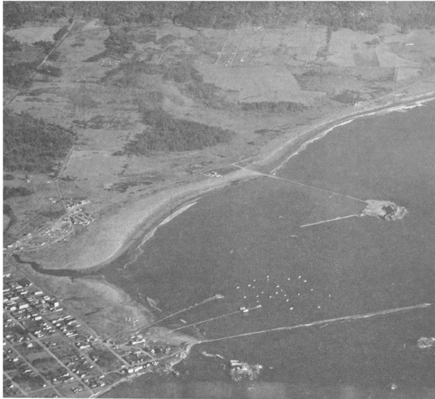
FIGURE 16. Crescent City Harbor. Photograph by the Waves Research Laboratory, University of California, November, 1946.
