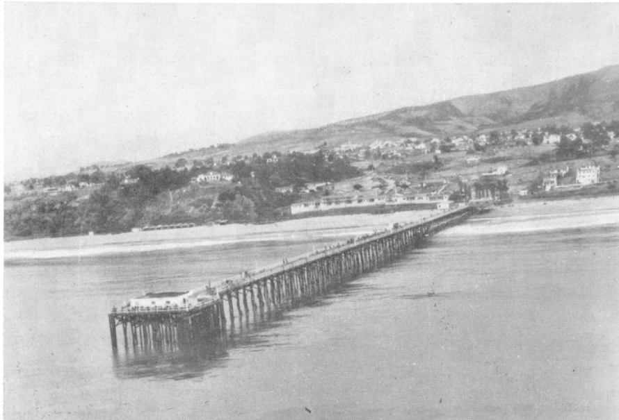
FIGURE 85. San Clemente and its pleasure pier. Photograph by R. D. Collyer, April, 1949.
