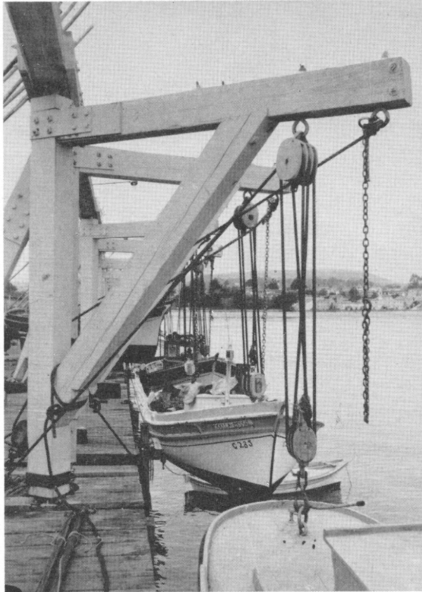
FIGURE 43. Fishing boats hoisted on davits to the Municipal Pier at Santa Cruz. Photograph by R. S. Croker, April, 1930.
