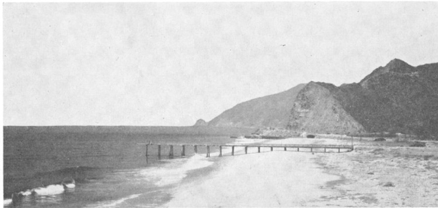
FIGURE 67. Damaged pier at Big Sycamore Creek Beach. Photograph by the Waves Research Laboratory, University of California, July 1, 1949.
