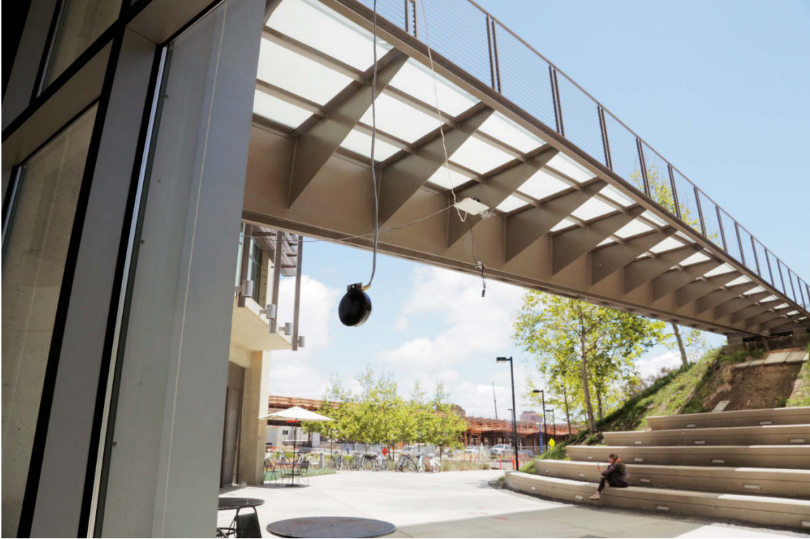
Figure 6. Window , installation view (interior), 2018.
