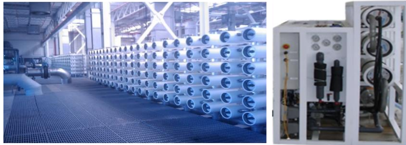
Fig. 1-3. (Left) Photograph of the desalination plant at Orange County, California (Capacity of 378,000 m 3 /day) [18], and (Right) a small mobile RO desalination plant (capacity of 45.4 m 3 /day) [19, 20]. The same size membrane elements (8”) are used in both plants demonstrating the scalability of RO desalination.
