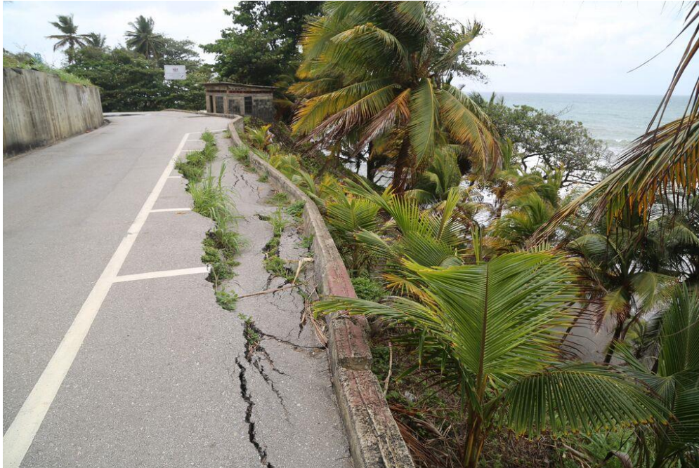
Figure 17. Sliding shoulder in Matelot
