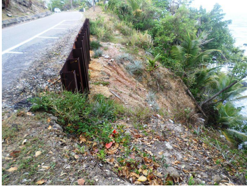
Figure 20. Protective structure to prevent sliding
