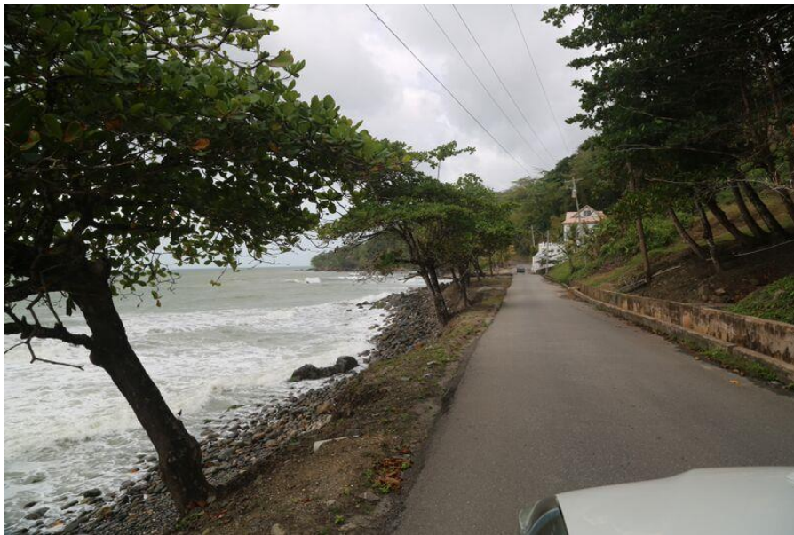
Figure 16. Road running adjacent to ocean in Matelot
