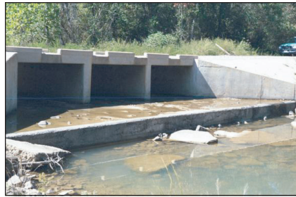
Figure 6. Bear Creek box culvert with drop. Figure 7. Muddy Gibbs crossing without a drop.
