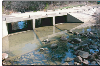
Figure 6. Bear Creek box culvert with drop. Figure 7. Muddy Gibbs crossing without a drop.
