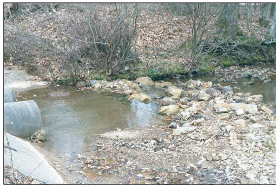
Figure 5. Vented low-water ford modified.
