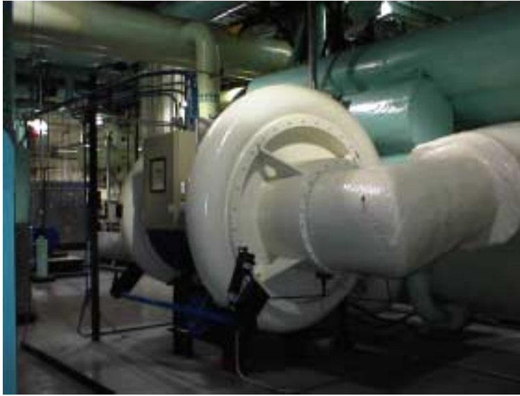
Figure 13 Centrifugal Chiller
