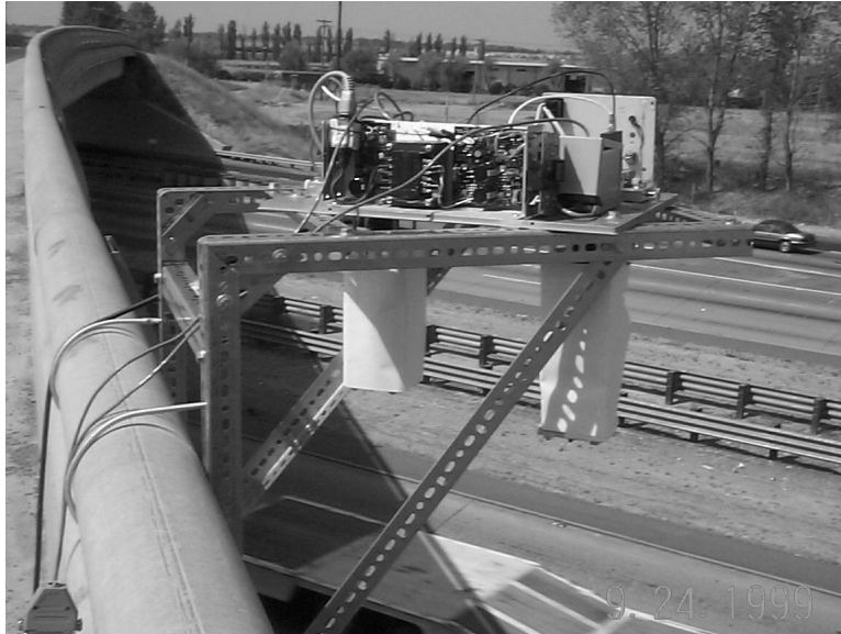
Figure 4.3: Detection system mounted above the highway
