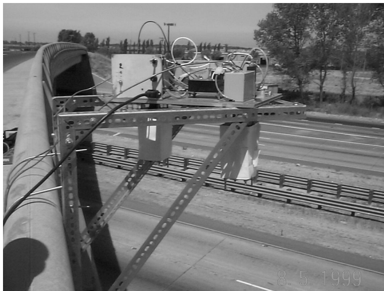
Figure 2.11: Testing prototype mounted on the cantilevered frame
