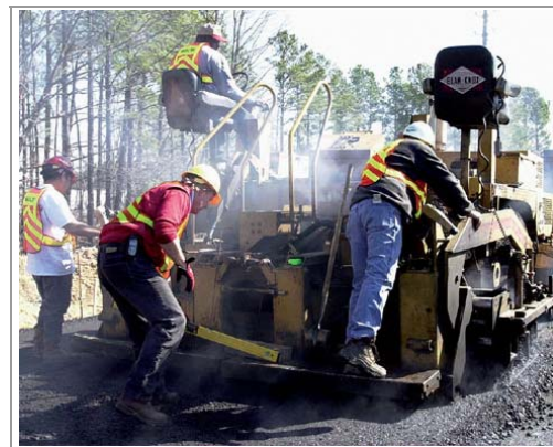
Figure 16 – Roadway paving emissions
