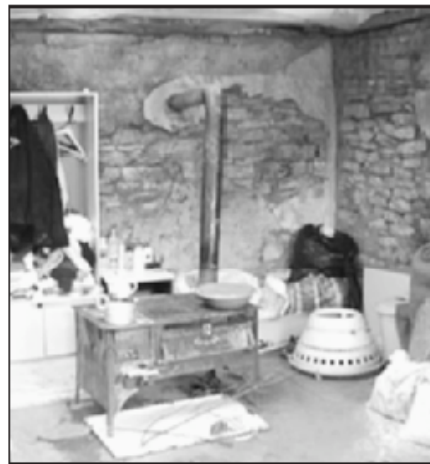
Figure 34. USAID "Warm-Dry Rooms" Project
