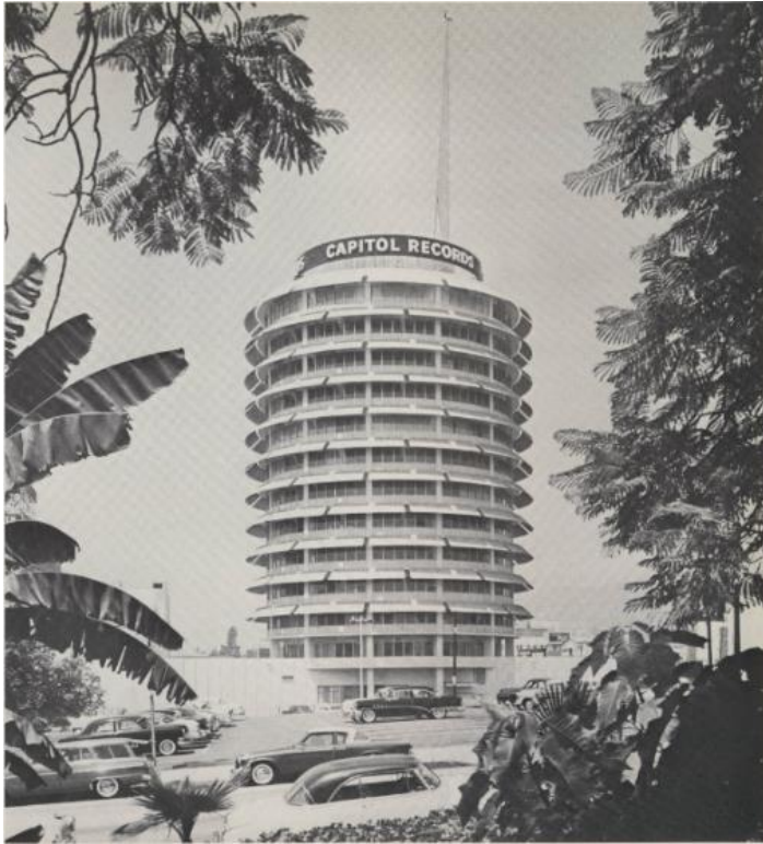
Figure 1.1: Capitol Records Tower. Image from Chris Nichols, ed., Built by Becket (2003), 27.
