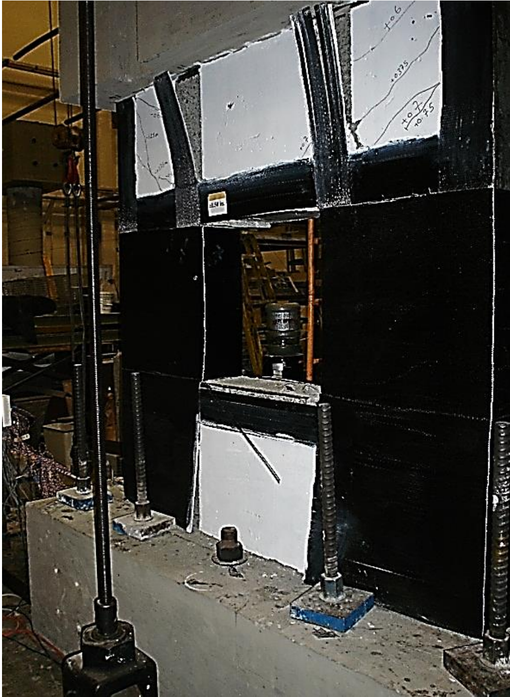
Figure (13): Failure of Wall Specimen (R-WO)
