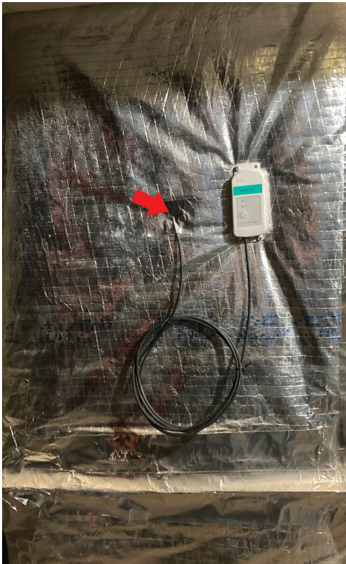
FIGURE 5 (left). Monitoring temperature and relative humidity at air handler supply duct. FIGURE 6 (right). CO 2 monitor. DAVID BITTERMANN
