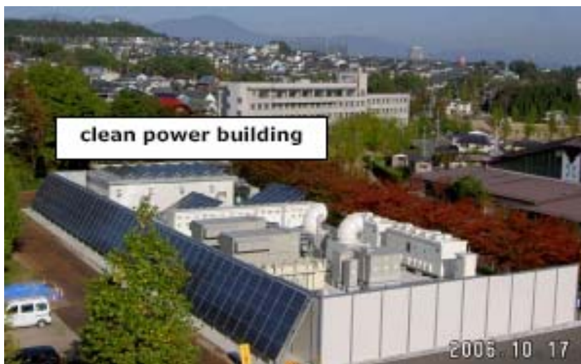
Figure 9. The Sendai Multiple SQRA Microgrid Demonstration
