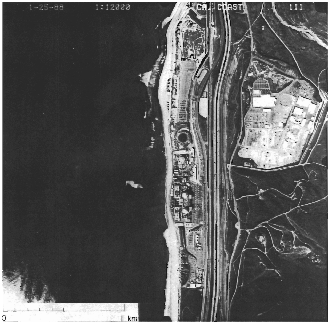
Figure 24. Aerial photograph taken 25 January 1988. Note much reduced beach width in front of Units 2 and 3 seawall. Contrast this with Figure 23.
