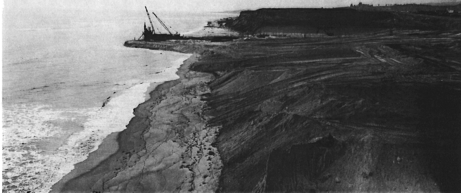
Figure 8. Photograph similar to Figure 6, but looking north from Station "B". Note the relatively narrow beach to the north of the construction activity. Also note the contact line between lower San Mateo sand formation and overlying terrace deposits in the exposed cliff cut.
