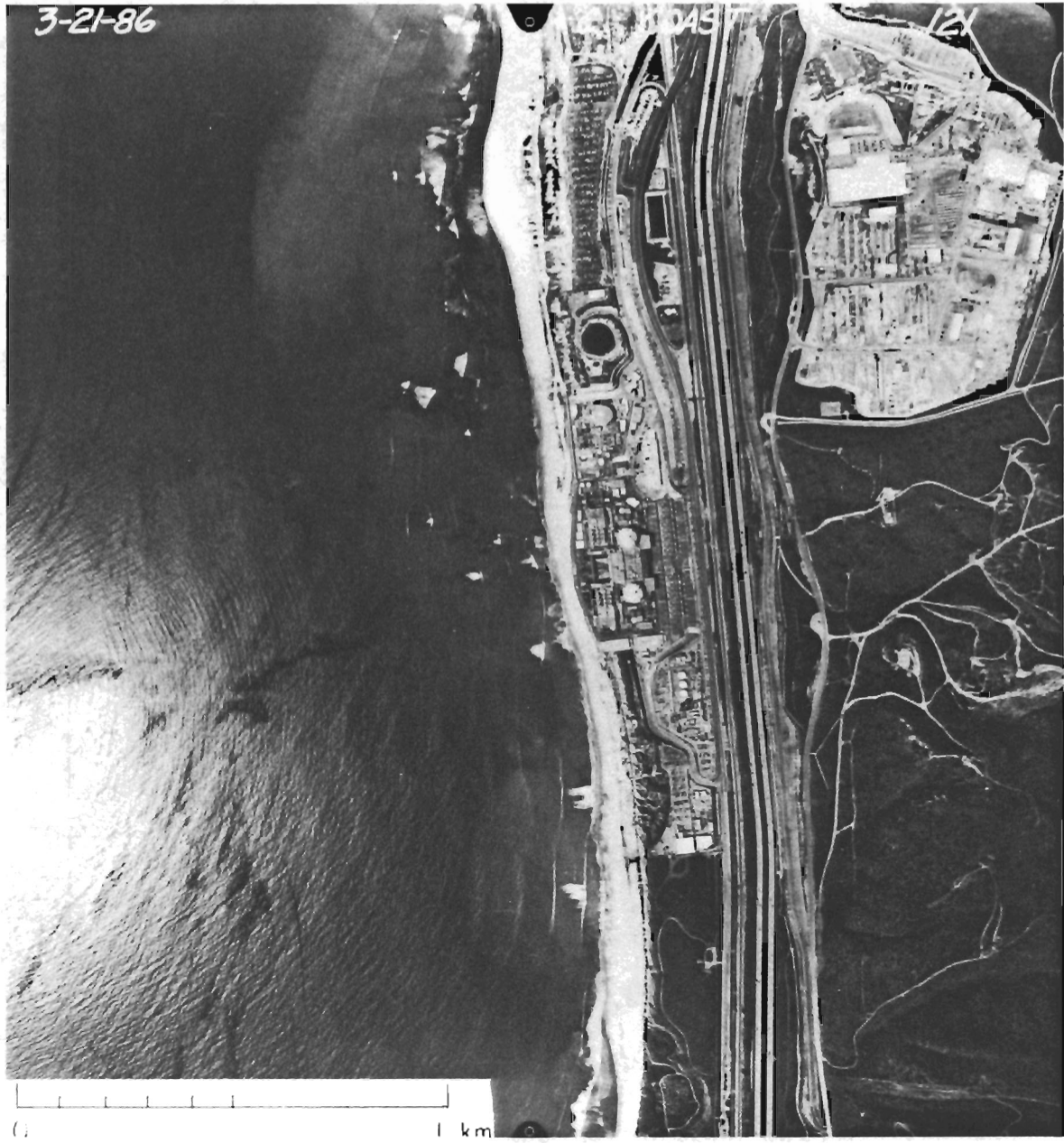
Figure 23. Aerial photograph taken 21 March 1986, about one year after removal of Units 2 and 3 laydown pad.
