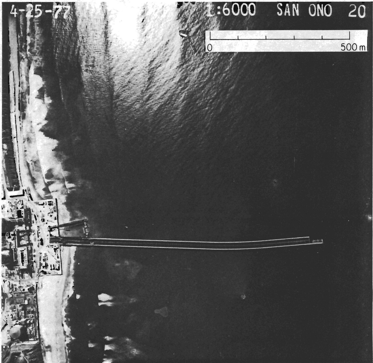
Figure 21. Aerial photograph of beach trestles used to lay Units 2 and 3 cooling pipes. Photo taken 25 April 1977. Note widened fillet beach upcoast of (below) laydown pad beginning to bypass the structure.
