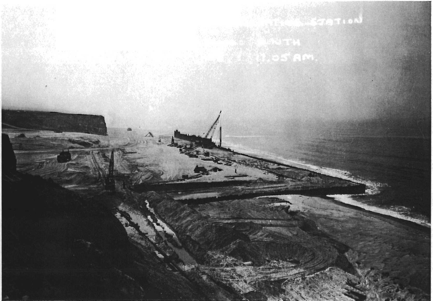
Figure 10. Photograph showing construction of Unit 1 laydown pad taken on 24 June 1964 from Station "A". Note sand spoil on north (foreground) side of sheetpile from continued excavations, in contrast to Figure 6.
