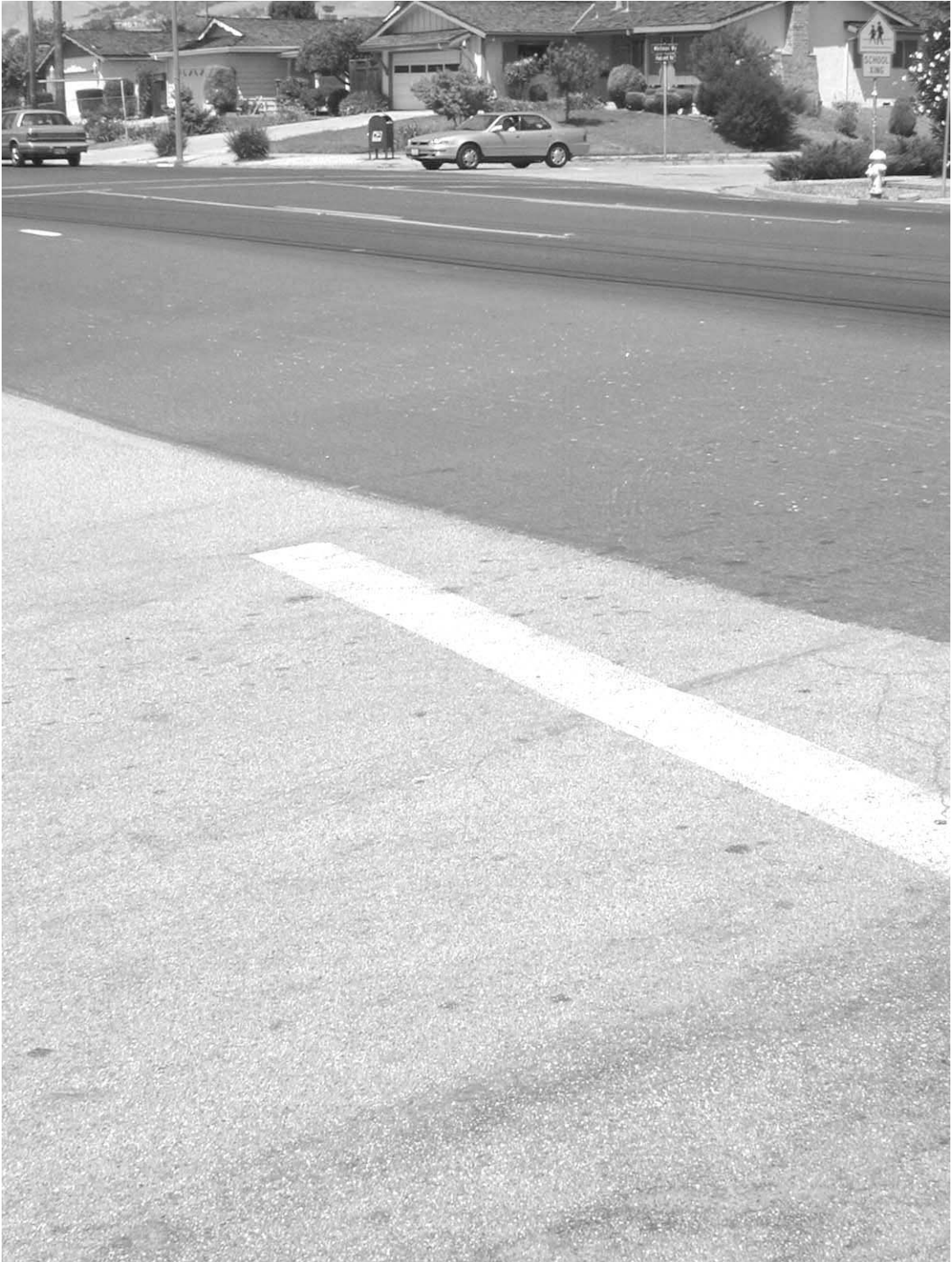
Fig. 8. Photograph of streets in San Jose, CA, that are paved with asphalt (in the middle) and chip seals (at bottom and top).
