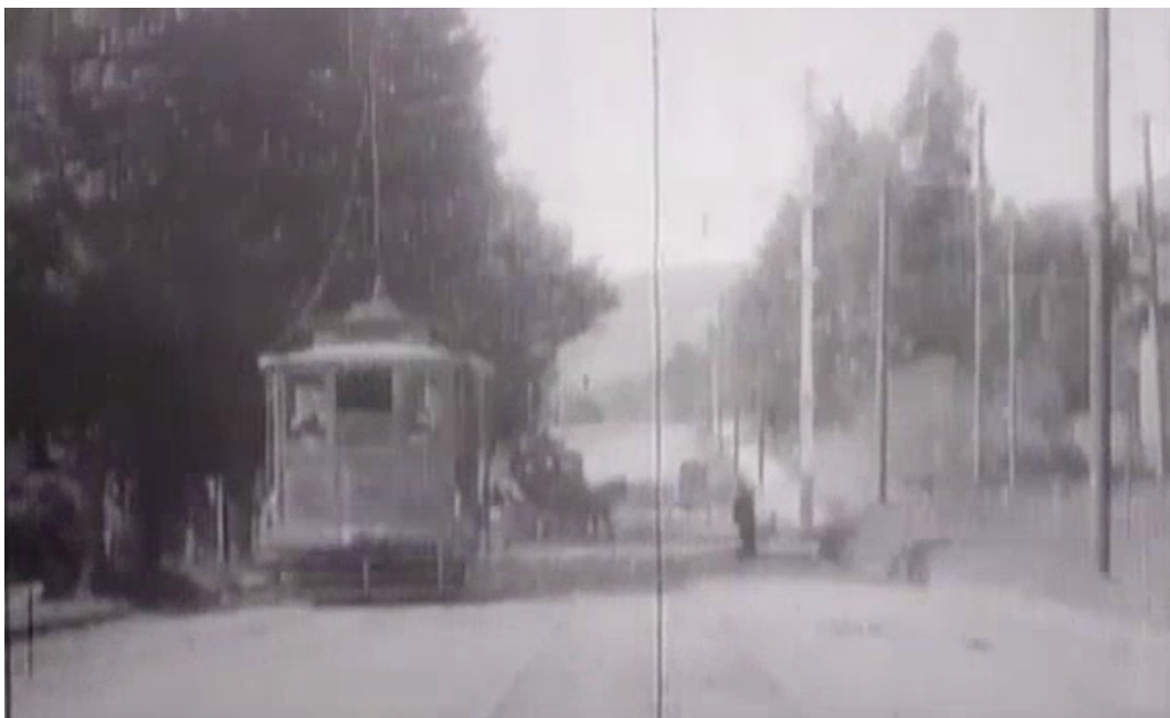
Figure 11. Streetcar line on Oxford Street. Source: Library of Congress, 1906
