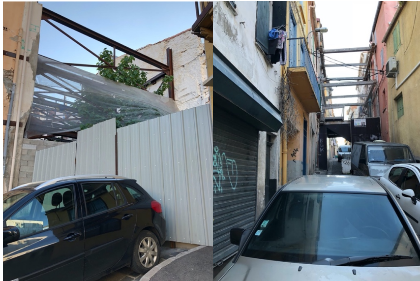
Support beams between buildings
